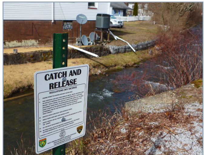
Figure 8. Straight pipes from homes and “catch and release” fishing sign on Elkhorn Creek.
