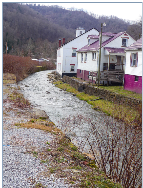
Figure 4. Straight pipes from residences into Elkhorn Creek.
