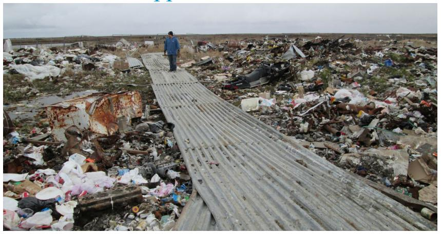
A drive through temporary metal road was built inside the dump fence.
