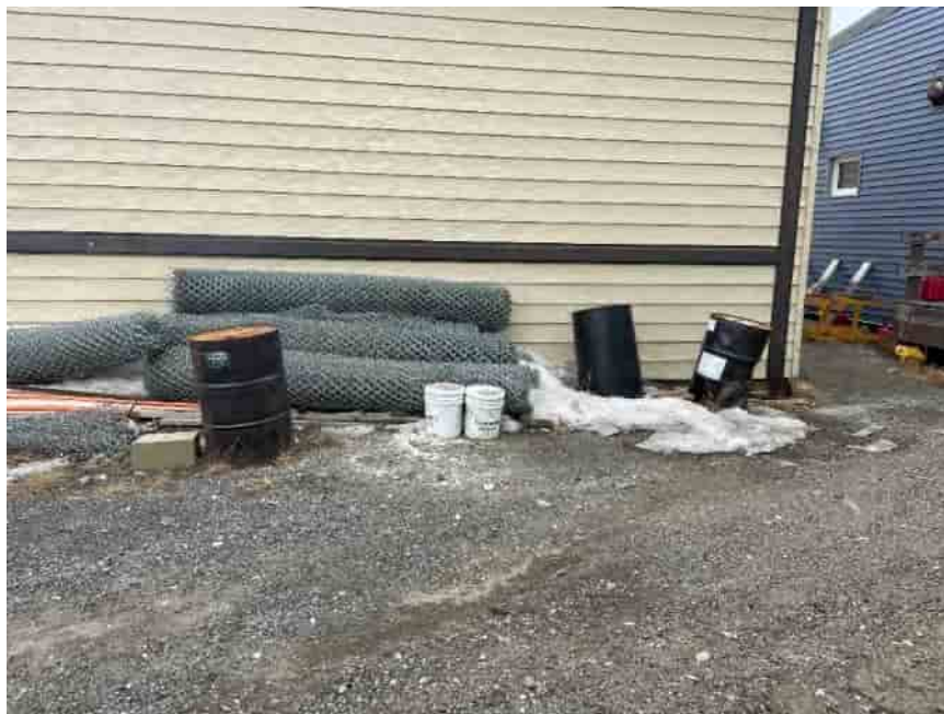
Photo No. 1 – HWMU-3, located south of the Warm Storage building, facing north. 8 June 2022
