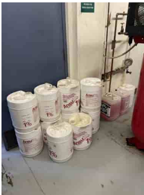
Photo No. 2 – Compressor wash and firefighting foam at SWMU-1. 9 June 2022
