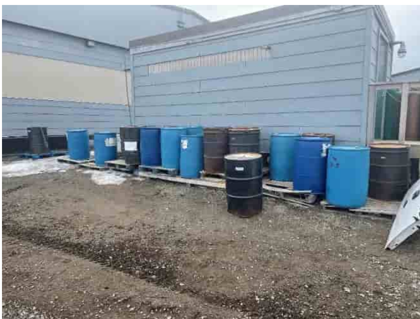
Photo No. 2 – HWMU-2, the transfer pumphouse northwest of the Bulk Tank Farm. 8 June 2022
