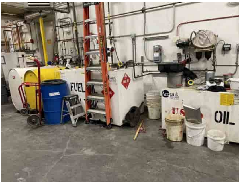
Photo No. 1 – SWMU-1 includes the interior of the entire Power Plant building. This unit contains only solid waste, including used oil removed from generators for regular maintenance. This photograph shows storage of fuel oil and used oil. 9 June 2022
