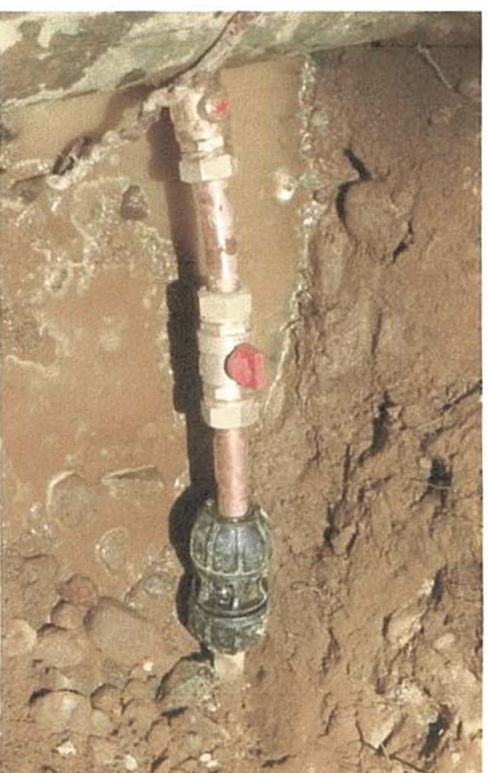
Installed new curb stop and copper tail piece
