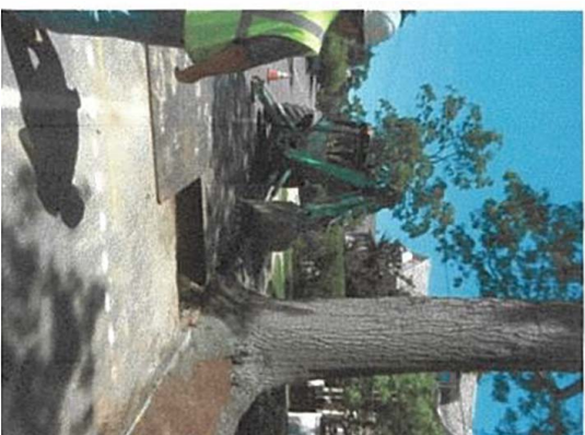
Access to main and for new curb stop
