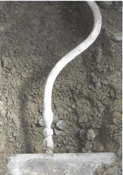
Existing lead service line at water main
