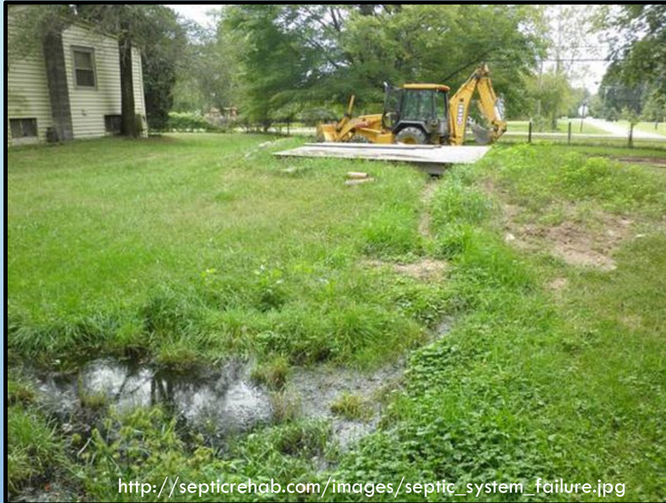
Failing septic system
