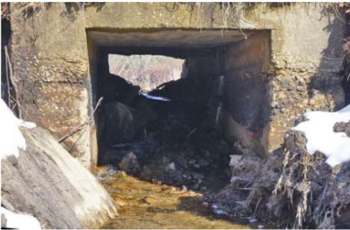
Clogged / Deteriorated Culvert
