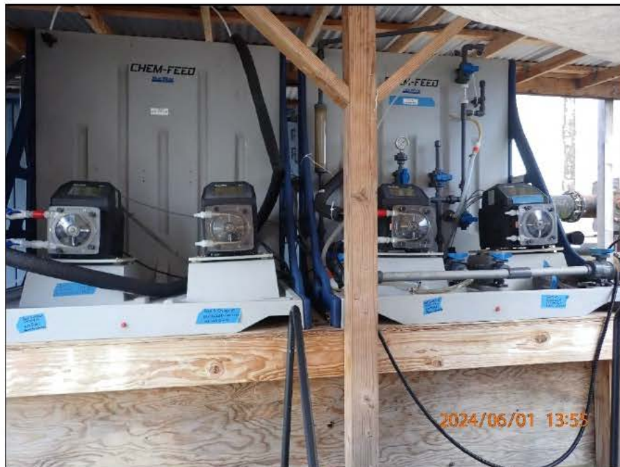
Photograph 4. The chlorine injection pumps were exposed to the outside environment.
