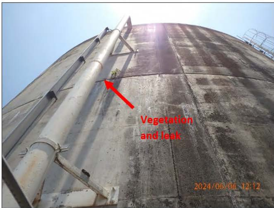
Photograph 10: Middle Tank had vegetation growth from a leak.
