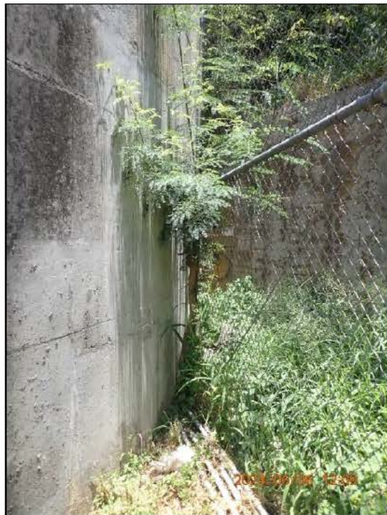
Photograph 8. Middle Tank had vegetation along the foundation, including a tree.
