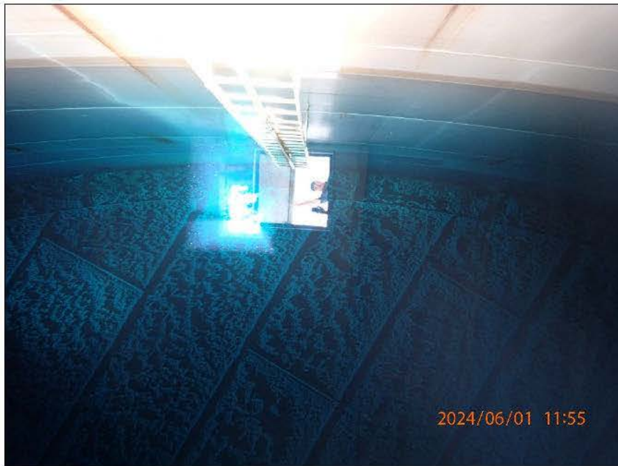
Photograph 10. JBPHH Date/Time Stamp is inaccurate. P6010032.JPG Description: [REDACTED] Sediment accumulation on floor.
