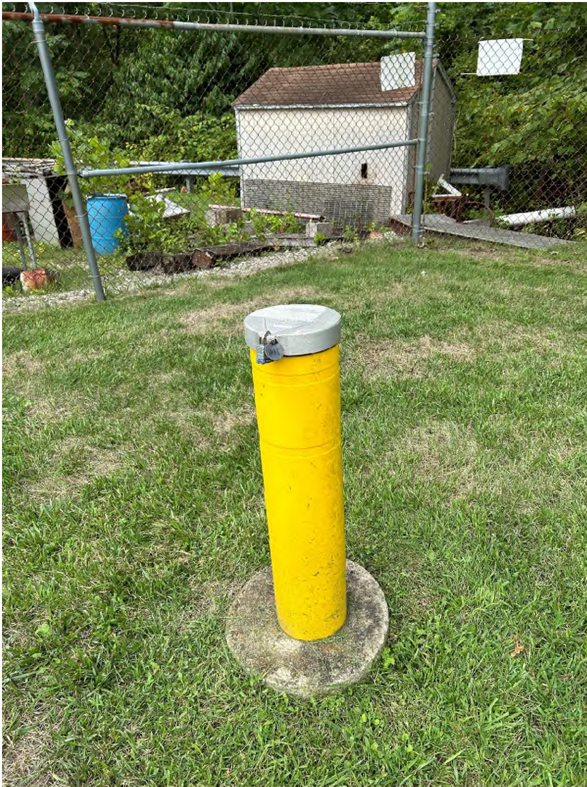
Figure 5: Close up of Monitoring Well MW-008.
