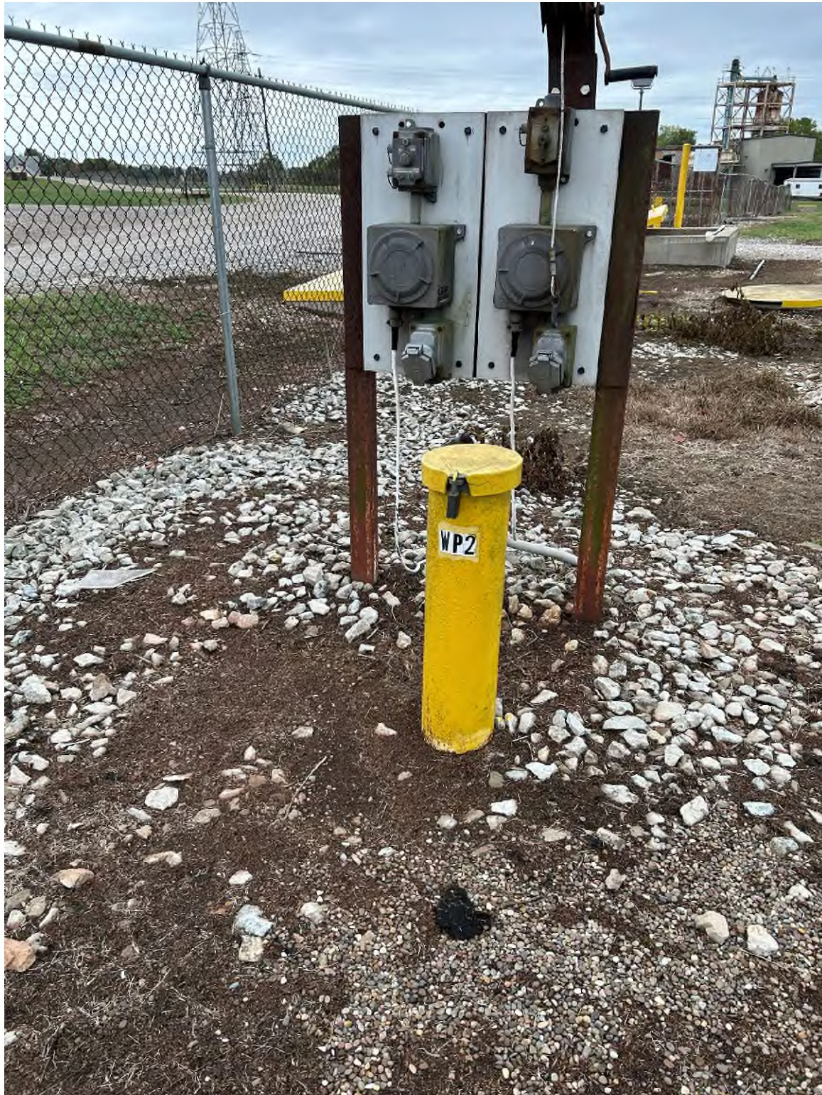
Image 7: The image of WP-2, one of ten (10) free product (oil) recovery wells in the vicinity of the oil ponds area.
