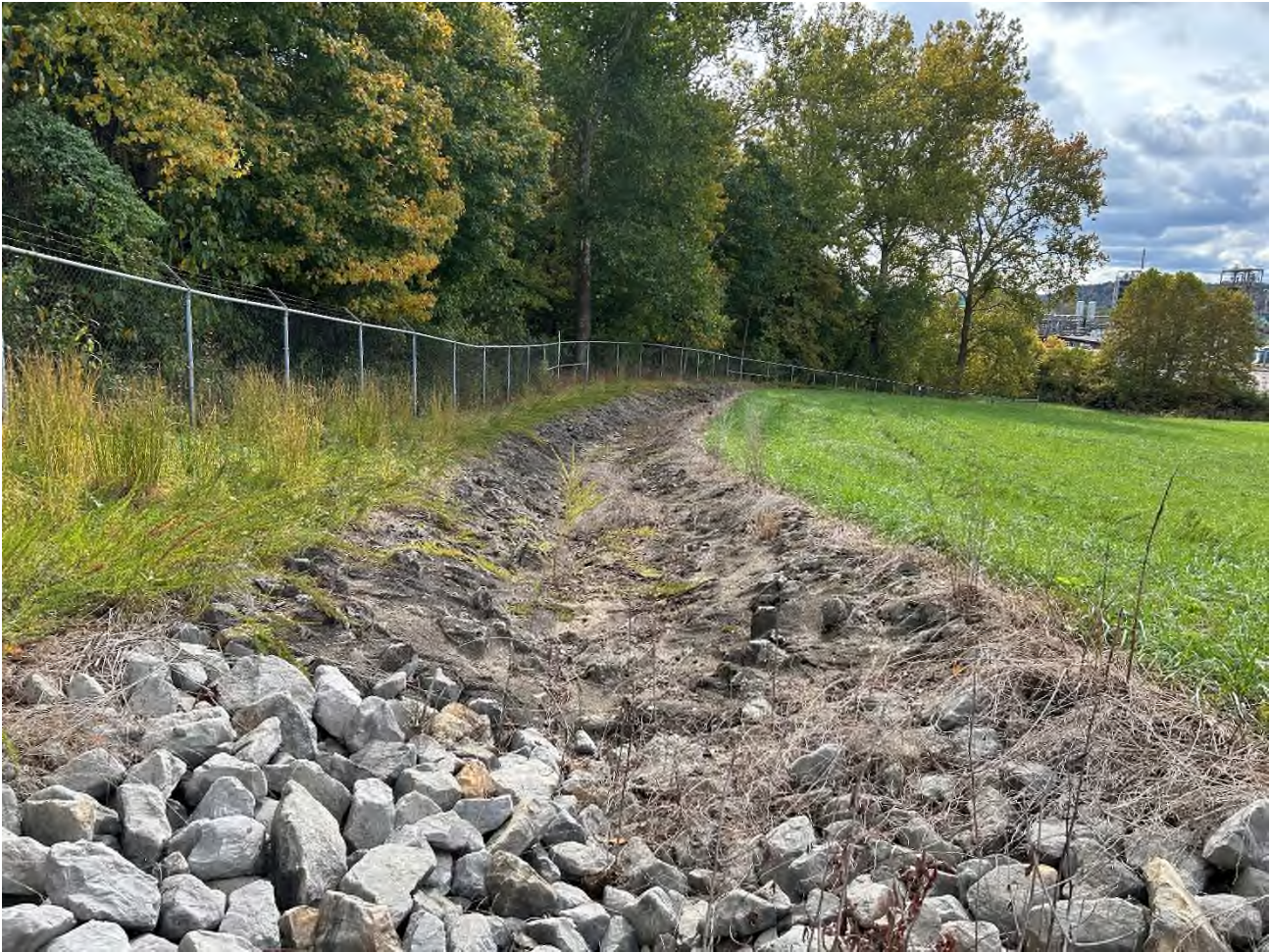
Image 1: Water/runoff diversion ditch near along the eastern boundary of the NIS, looking west/southwest.
