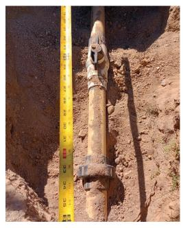
Potholing is an excavation method that involves digging small holes to identify the location, depth, and type of underground service lines.
