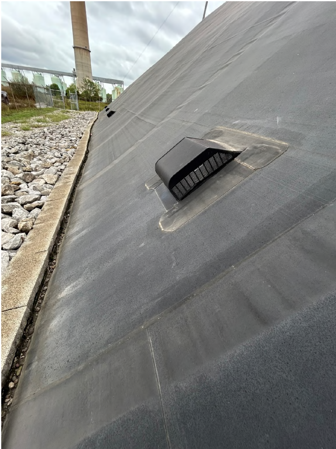
Image 10: Looking west along northern edge of the SPL Pile where the air vents are visible. Air vents were installed around the top and bottom perimeter of the wood substructure supporting the EPDM Cover. Also visible is the small rock/rip rap along the steep pile wall for water dissipation.
