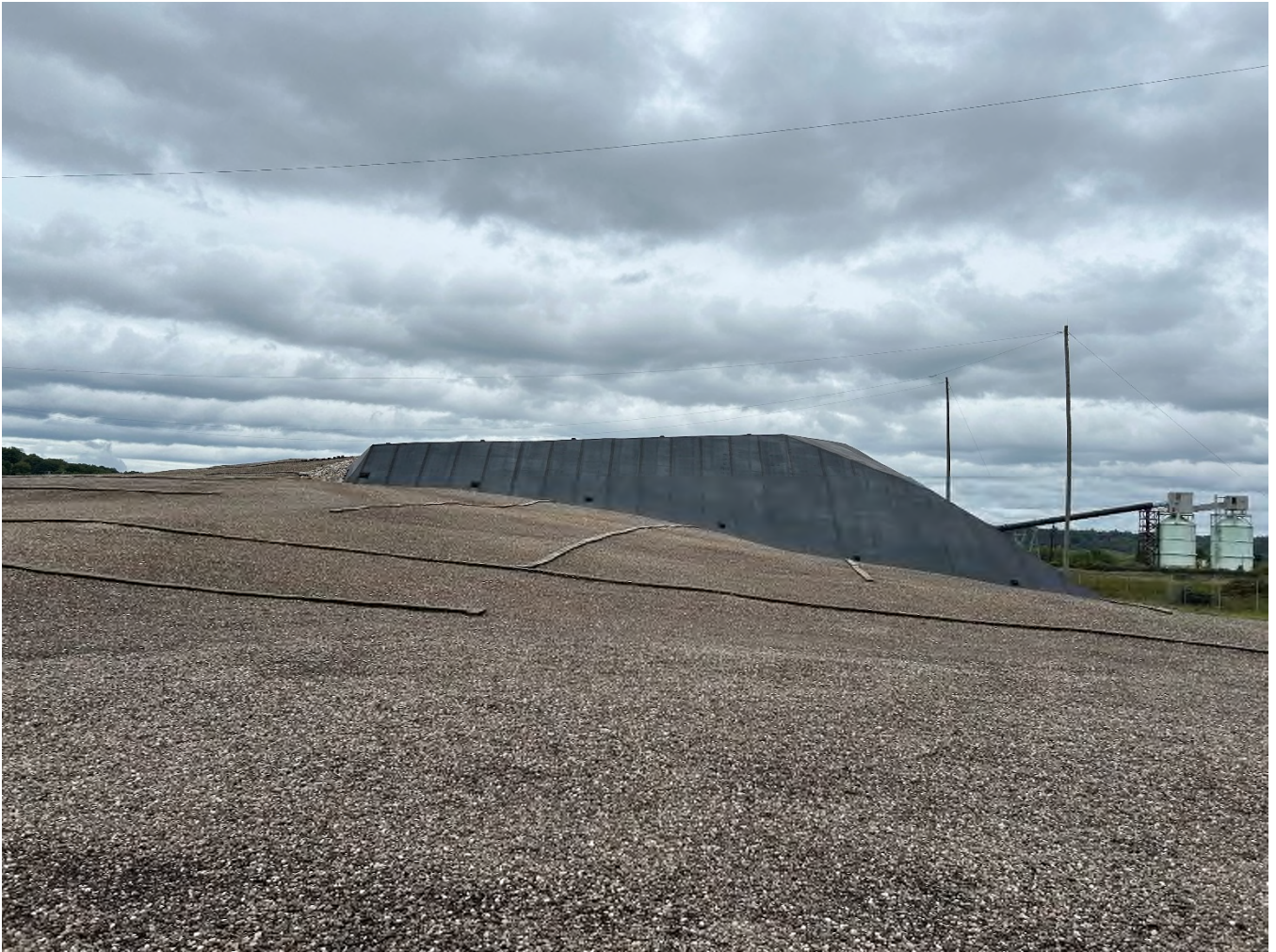
Image 5: Looking north near the southeastern corner of the SPL Pile; visible here the gravel covered gently sloping southeastern part and the southern half of the EPDM covered portion of the pile.
