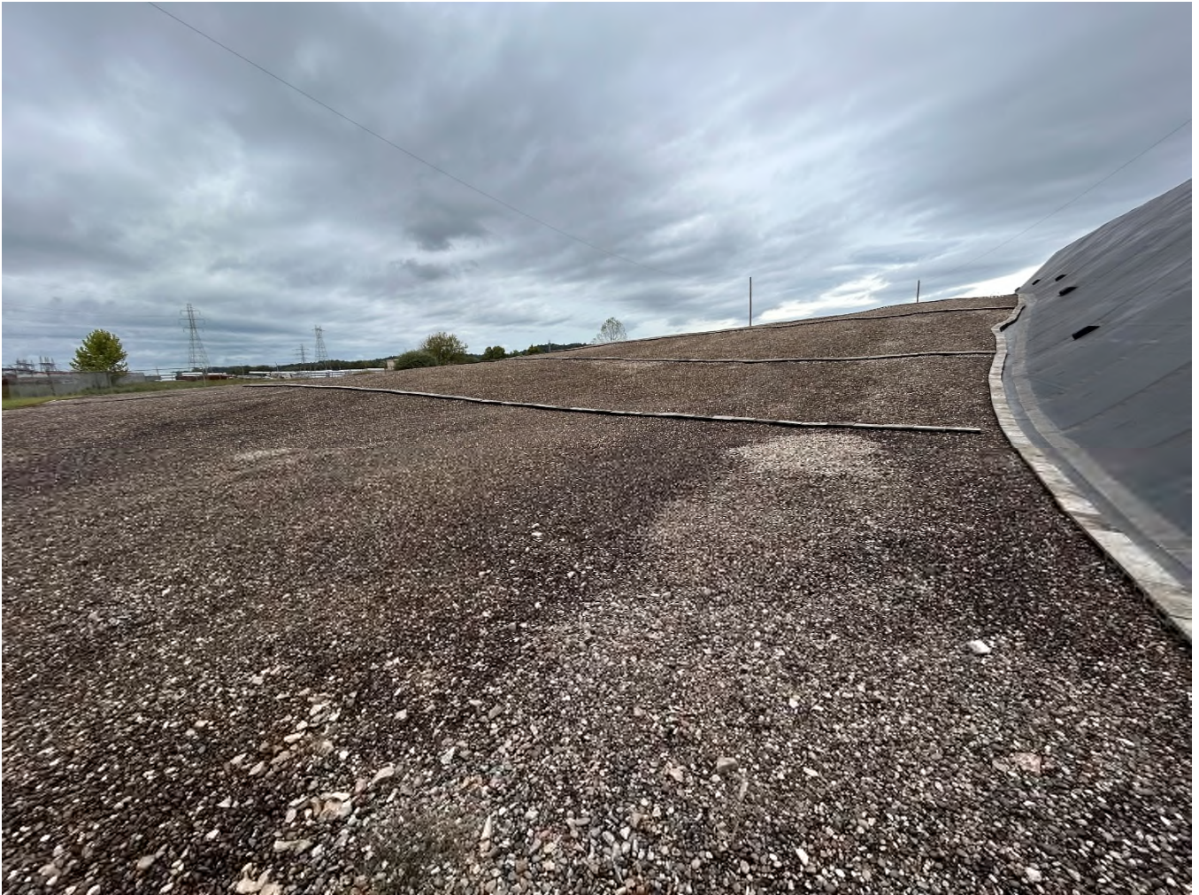
Image 4: Looking west near the mid-point of the eastern edge of the SPL Pile, where a steeply sloping EPDM cover goes under the gravel covering the less steep southern part of the pile. Linear features over the gravel are cinder blocks to walk and conduct inspections, and, if needed repair work.
