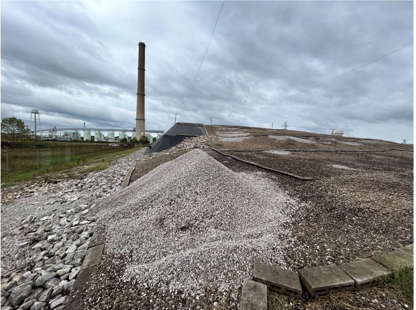
Image 8: Looking east near the northwest corner of the pile; river rock/gravel to use as fill between the washed out areas of the 4-6 inch rip rap rock at the foot of the SPL Pile. The 4-6 inch rip rap is used for water velocity reduction/water dissipation.
