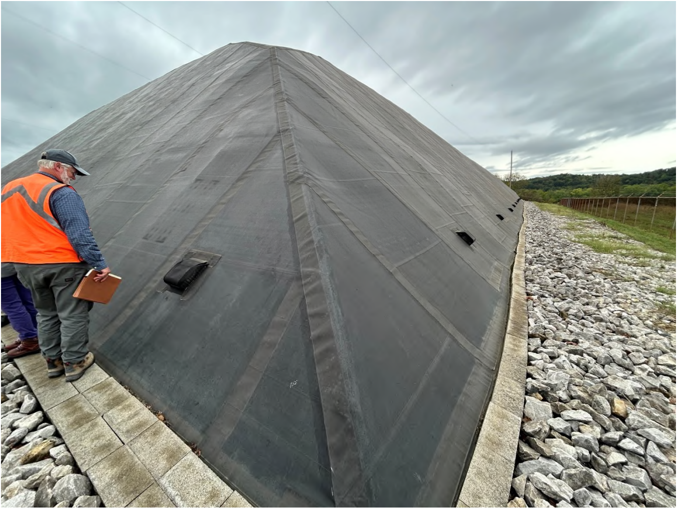
Image 1: A close look at the EPDM cover; looking east from the west corner from the SPL Pile.
