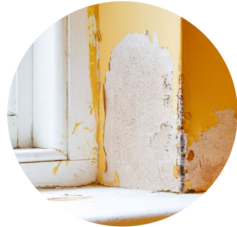
Lead-based paint deteriorates and creates contaminated dust and soil.
