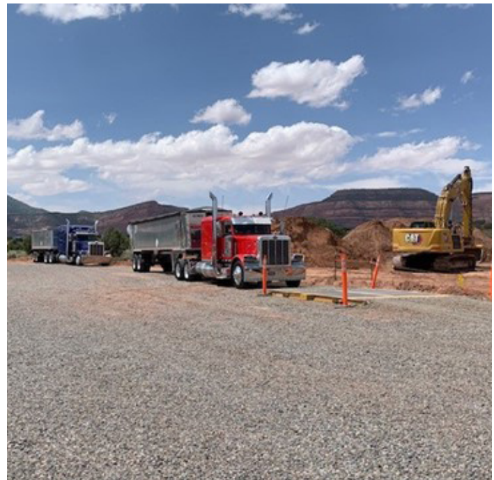
Trucks hauling soil off site during the 2023 Cove Transfer Station TCRA.
