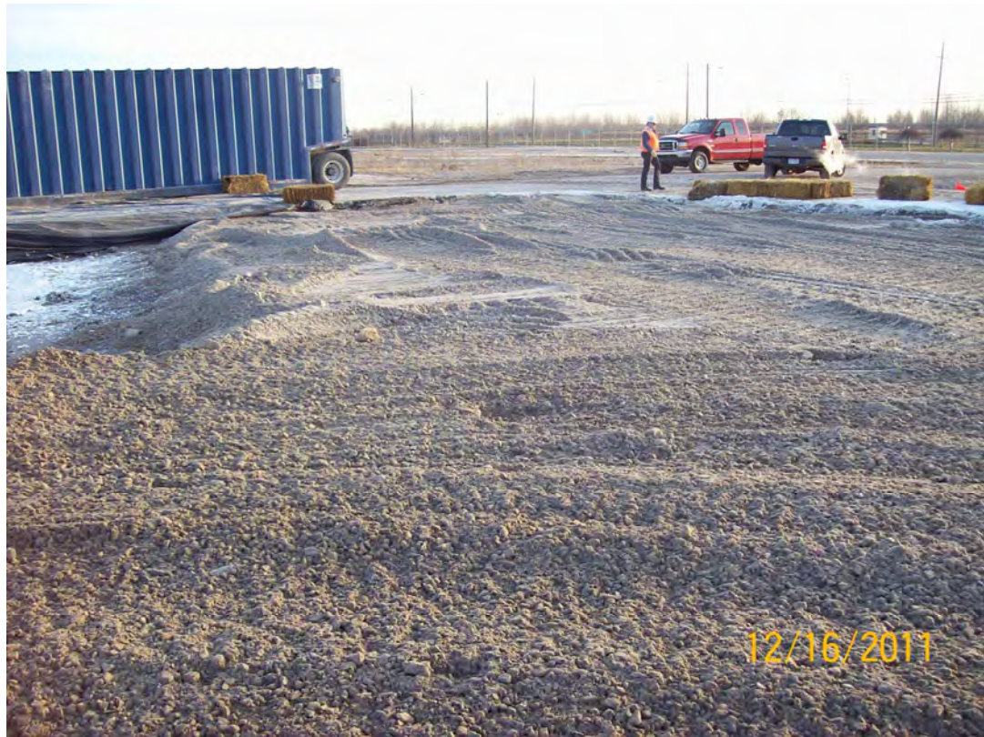
D11 Excavation backfilling & Gravel Capping operation (view – Northeast)
