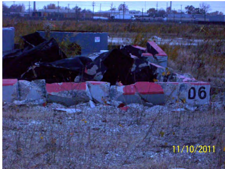
D6 Excavation- Above Grade Concrete Demolition (view West)
