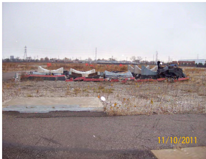
D3 Excavation- Above Grade Concrete Demolition (view West)
