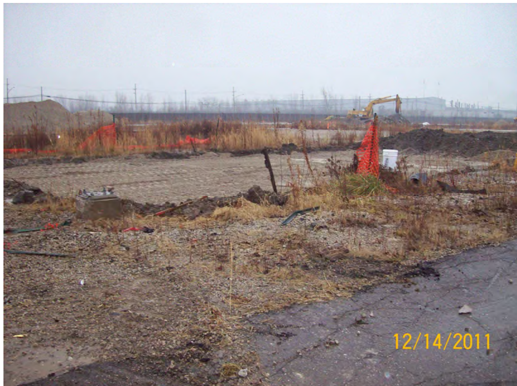
D34 excavation with backfill (view – Southeast)
