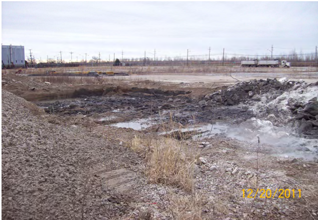
D34 Excavation with soil solidification (view – Northeast)
