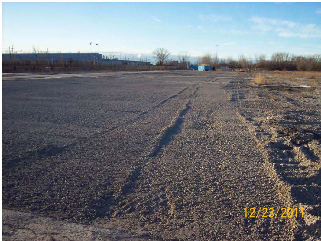
D3 through D11 excavations with Gravel Cap (view – South)
