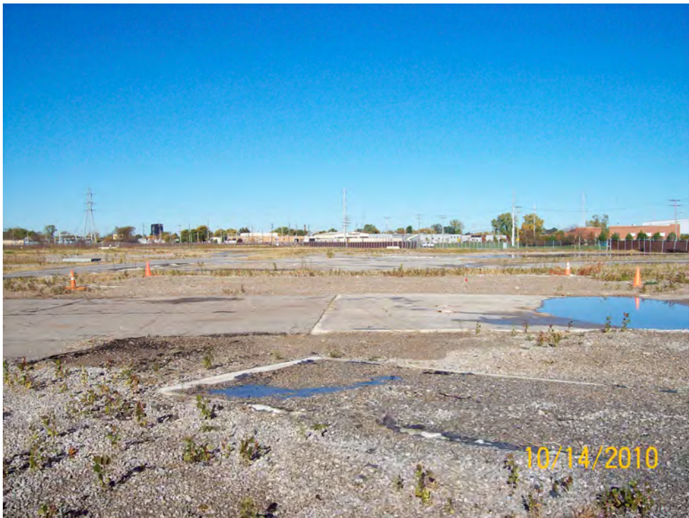
Photo 10: D34 Facing West (demarcated by cones)
