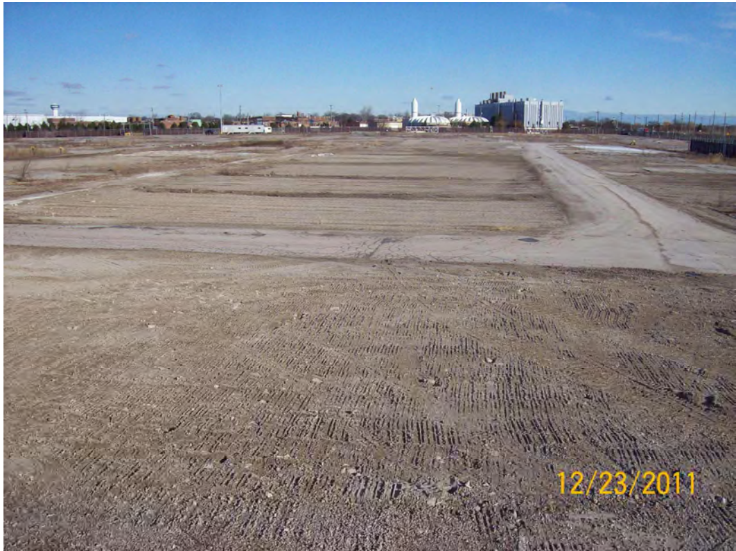
D2 through D11 Excavations with Gravel Cap (view – North)
