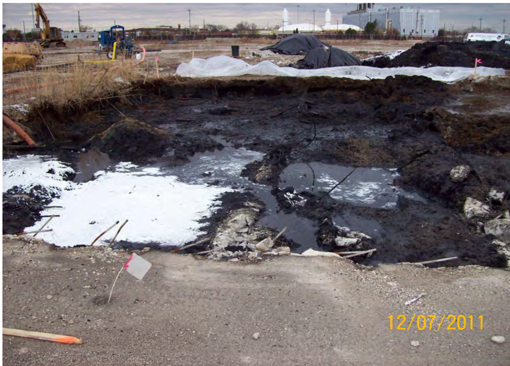
D10 Excavation with odor suppression foam (white) (view – North)
