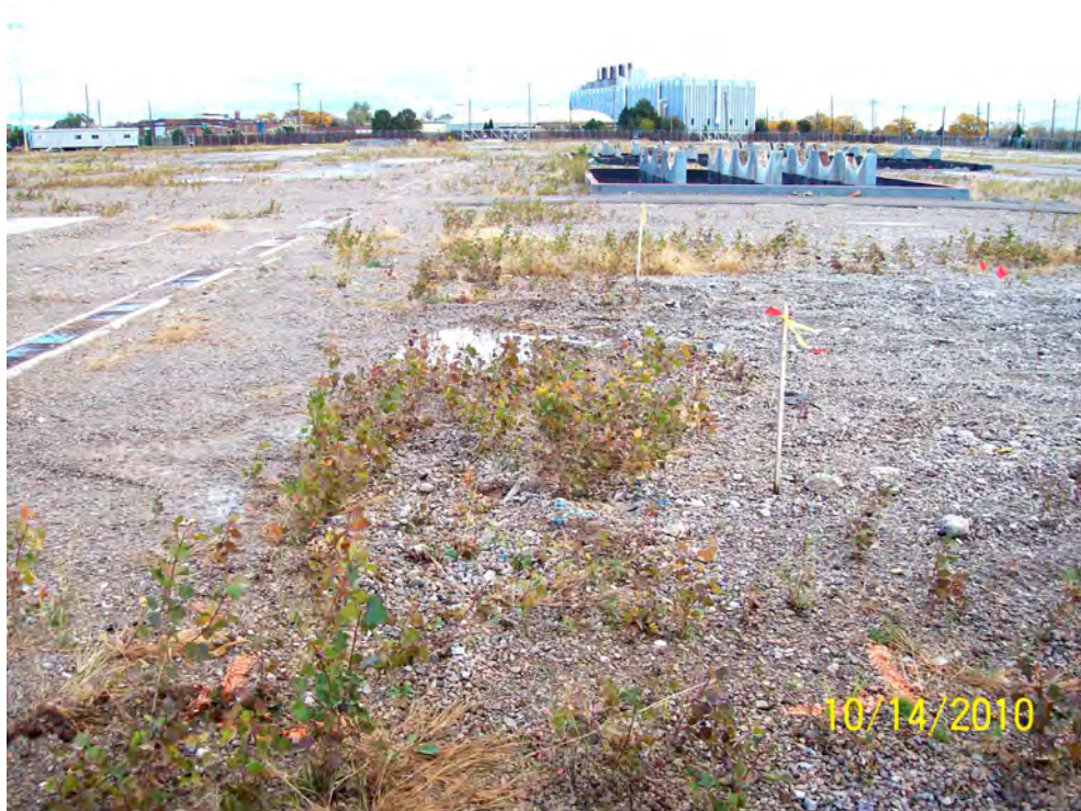
Photo 6: Excavation Area West of D8 (demarcated by paint marks)
