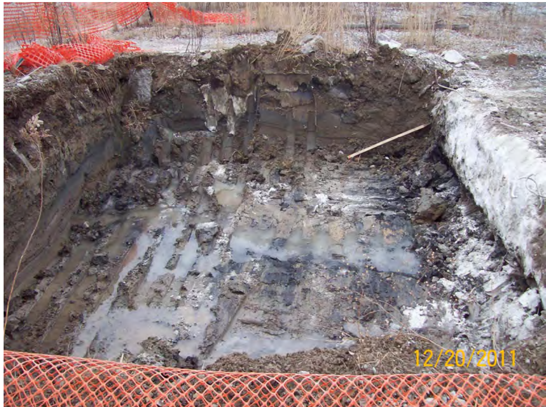
SB-16 Terminus of Excavation (view – North)
