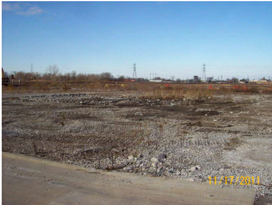
D11 Excavation- Post- Above Grade Concrete Demolition (view southwest)
