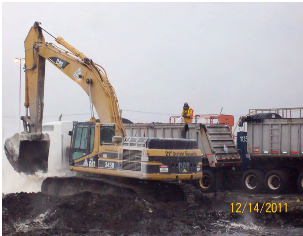
Soil solidification operation & Transport odor suppression application (view – Northwest)
