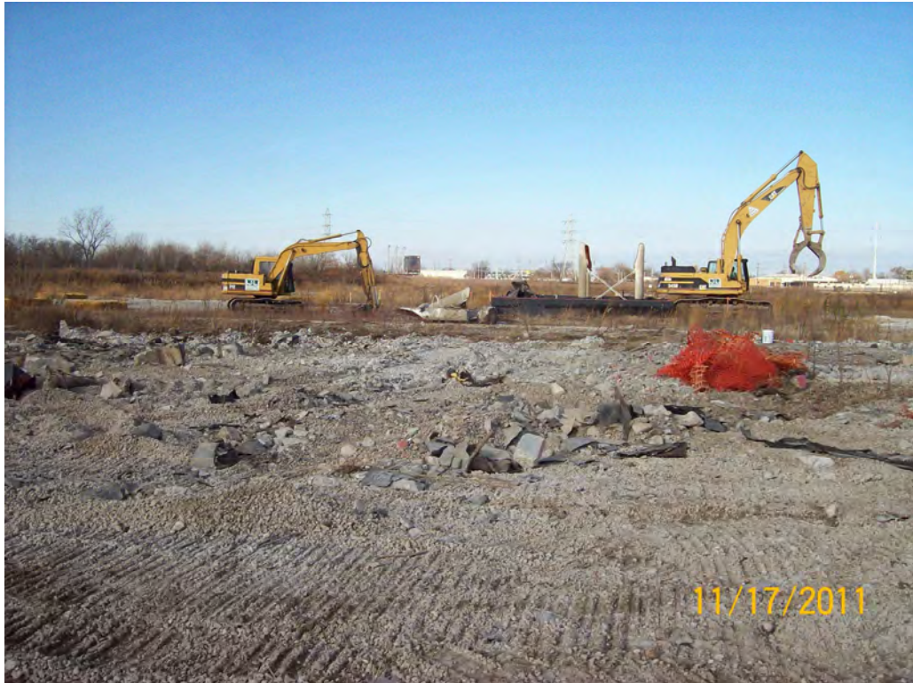
D5 D30 excavation (foreground) D42 excavation with concrete pillars (background) (view- West)
