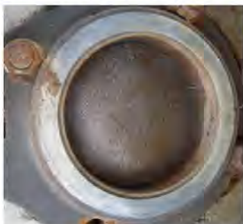
The best design is to install the #24 mesh screen between two flanges.
