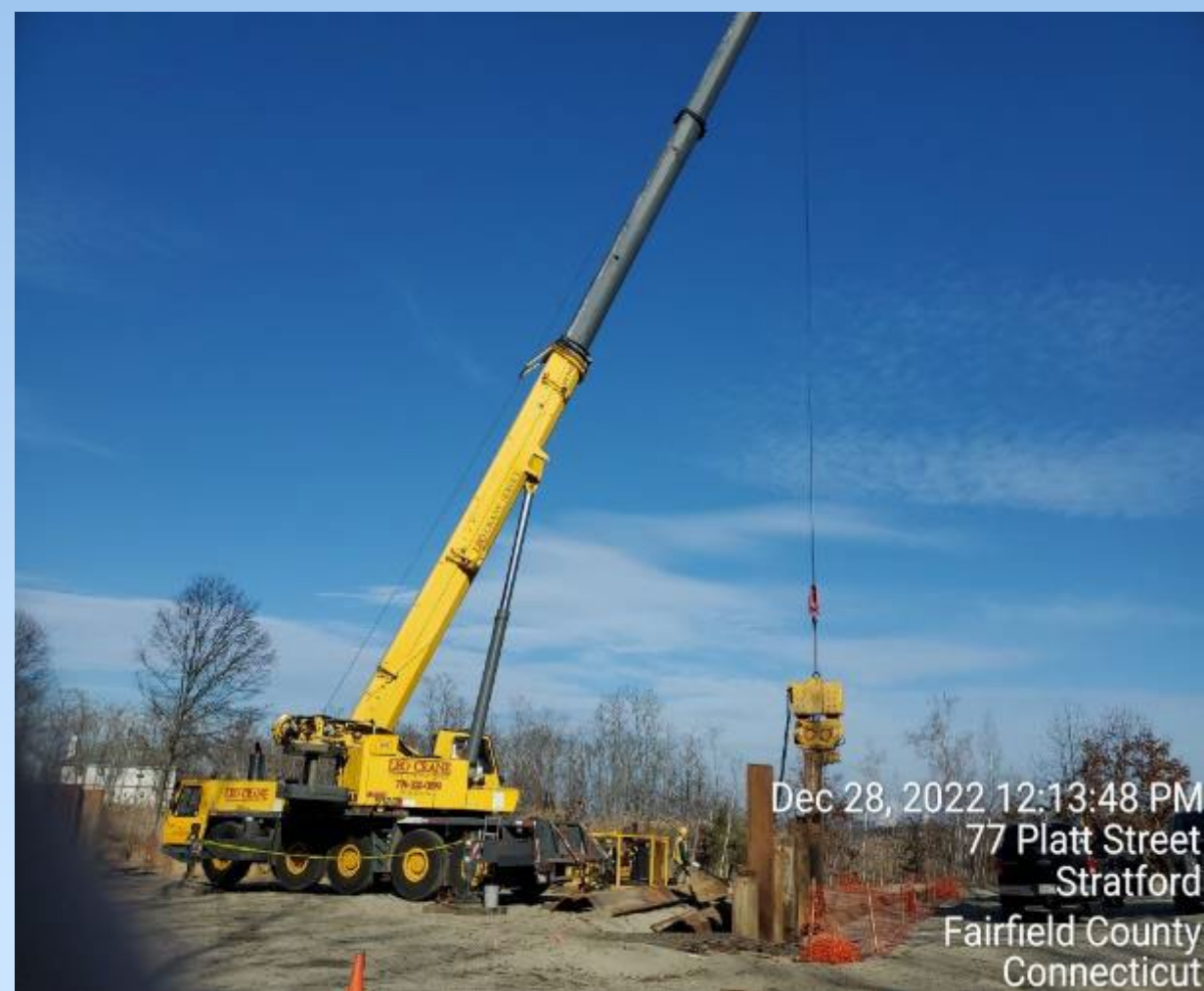
Sheet pile installation
