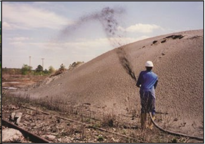
Application of Posi-Shell® via Extension Hose
