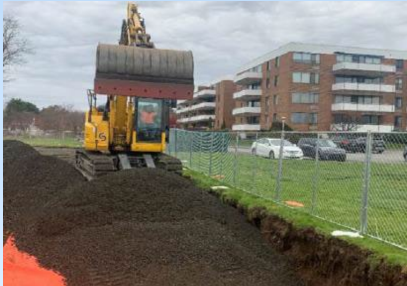
Beacon Point- Placing Clean Fill
