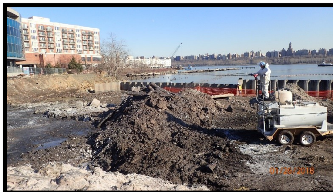
Worker applying Posi-shell.
