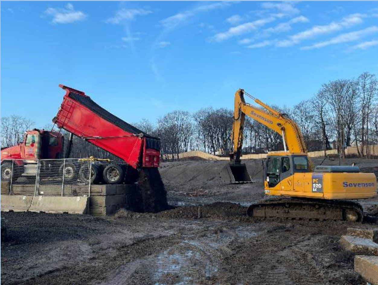
Material Placement Within OU4 Consolidation Area
