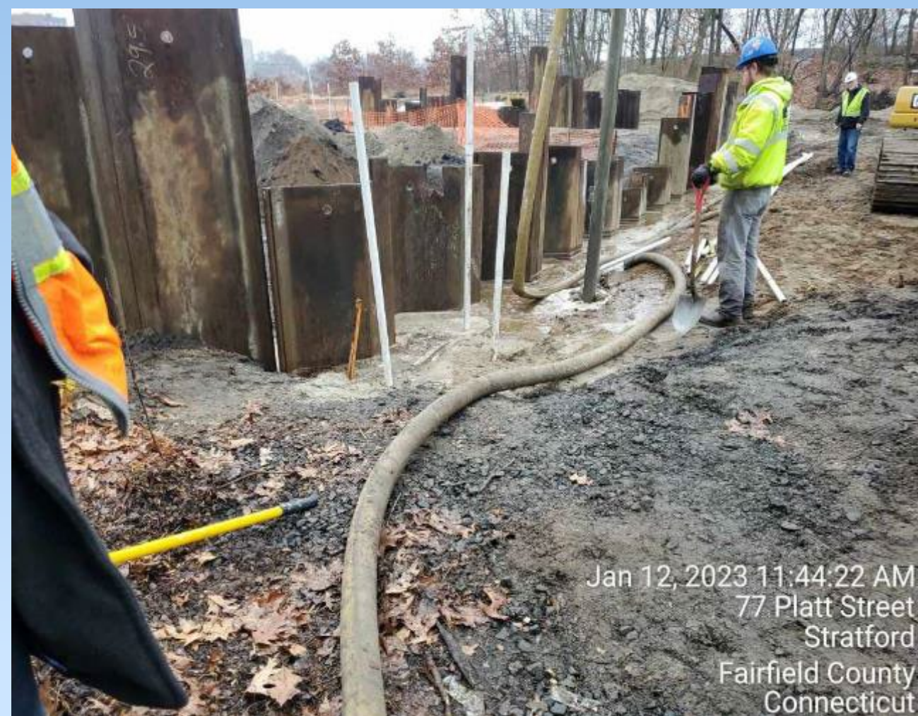
Dewatering well point installation
