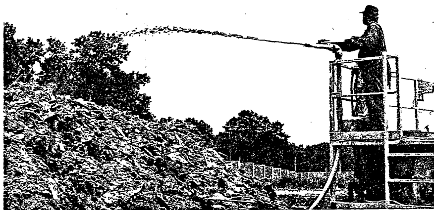
Figure 20. Application of Posi-Shell™ slurry with spraygun mounted on mobile sprayer.
