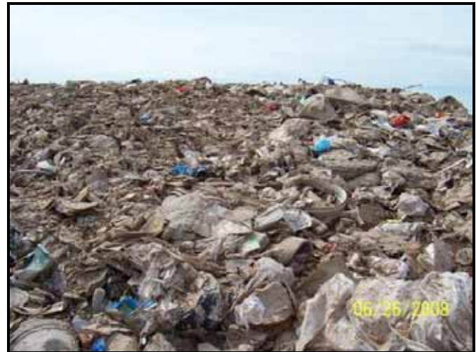
Example of inadequate application of cover material
