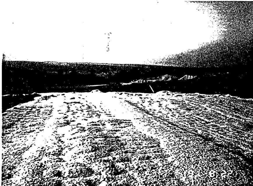
Figure 5. RUSMAR® foam immediately after application of a 6-in. (15-cm) thick layer.
