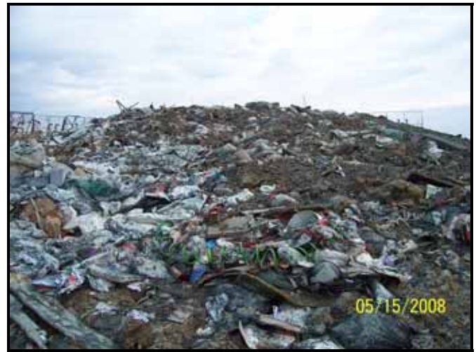
Example of inadequate application of cover material
