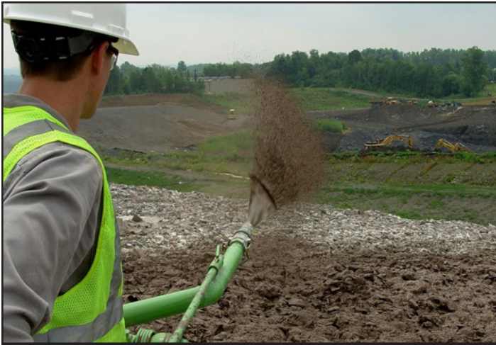
Application of Posi-Shell® via Deck-Mounted Discharge Wand
