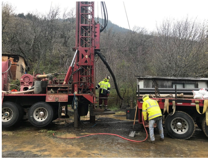
Drilling for the new drinking water source wells at the BIA Cooks-In-Lieu site
