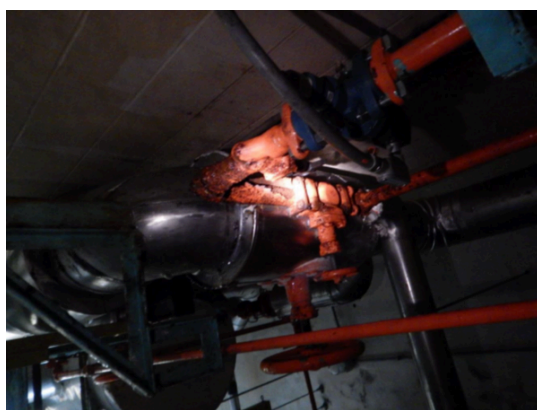
A corroded pipe at an Anheuser-Busch Facility leaking anhydrous ammonia
