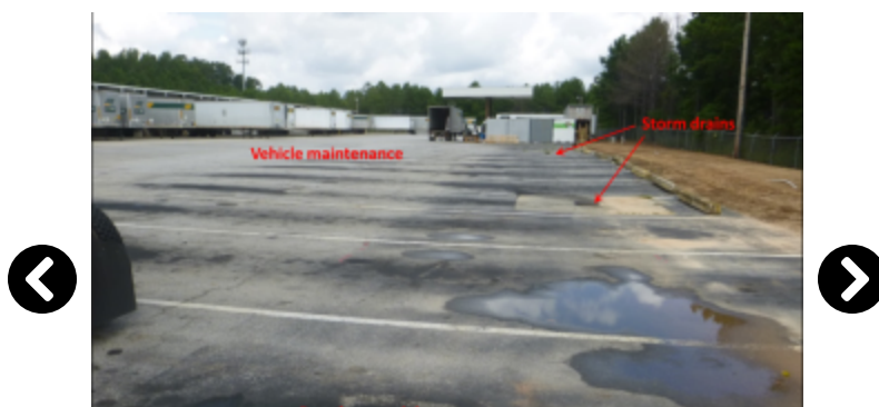
Petroleum product stains and residue due to vehicle maintenance which will flow into the nearby storm drains.
