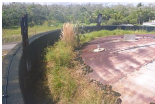
Severe corrosion at the sludge processing tanks has caused unsafe conditions, preventing maintenance of roof and causing further corrosion at Hilo Wastewater Treatment Plant
