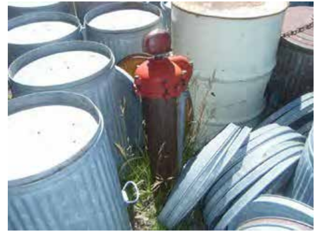
Potential sources of contamination surrounding wellhead
