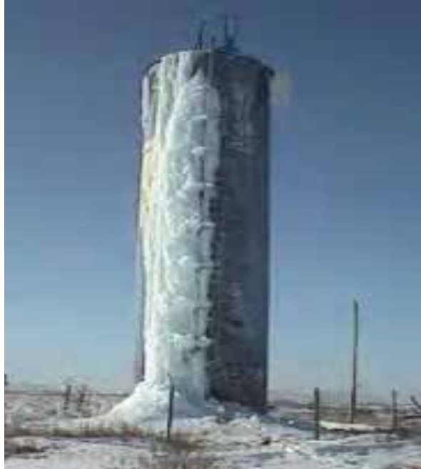
Frozen finished water storage tanks
