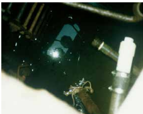
Dead snakes and mice floating in a spring box
