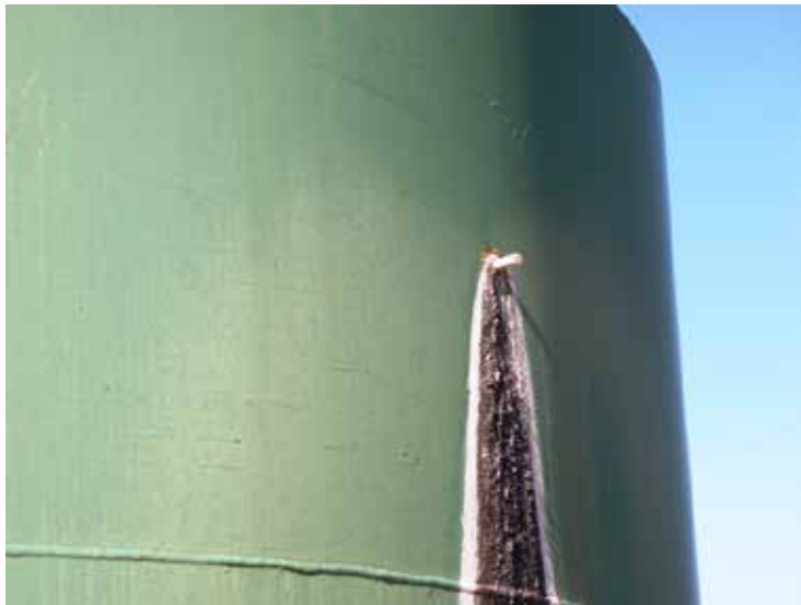
Un-repaired bullet hole in storage tank.
