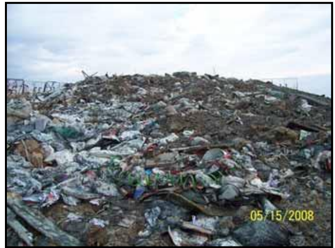
Example of inadequate application of cover material
