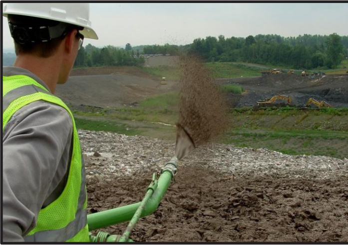
Application of Posi-Shell® via Deck-Mounted Discharge Wand
