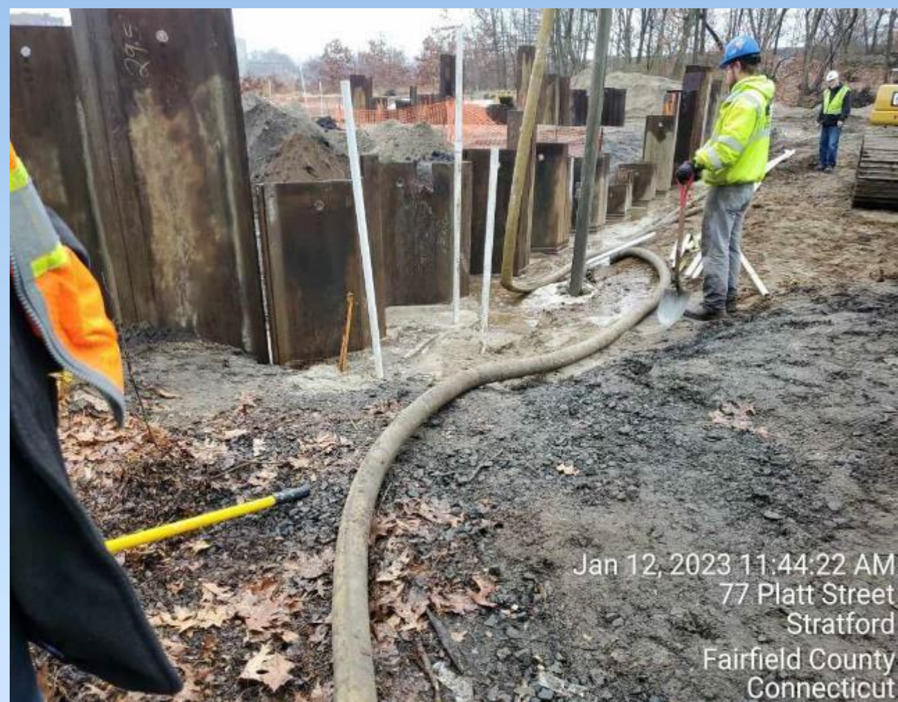
Dewatering well point installation
