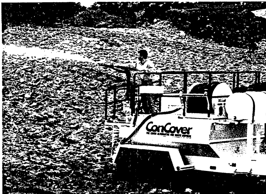
Figure 16. Application of ConCover® slurry onto a working face using trailer-mounted CAPS.
