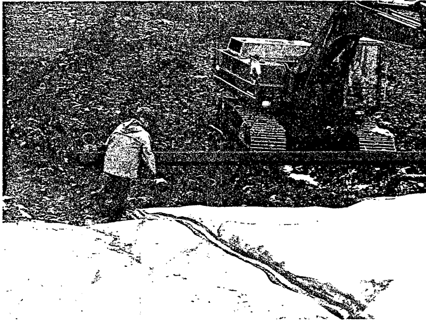
Figure 25. Trailing edge of panel being detached from lifting bar after extension over working face.
