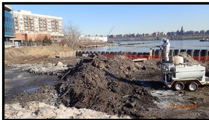
Worker applying Posi-shell.
