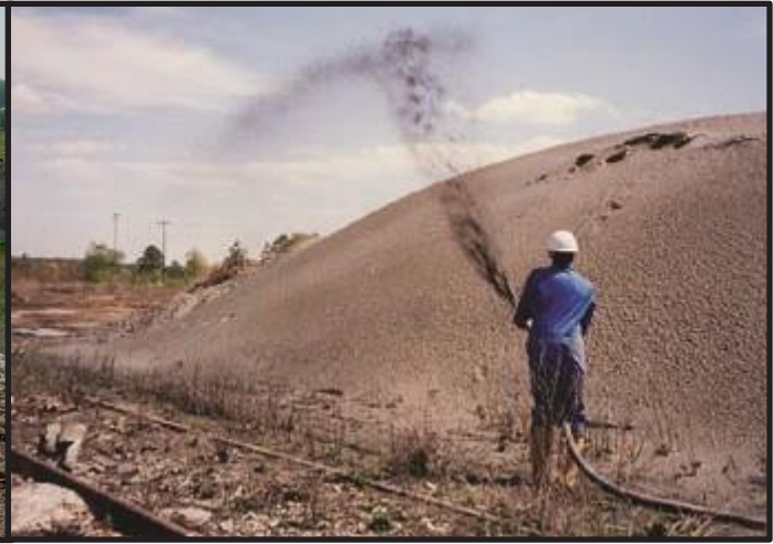
Application of Posi-Shell® via Extension Hose
