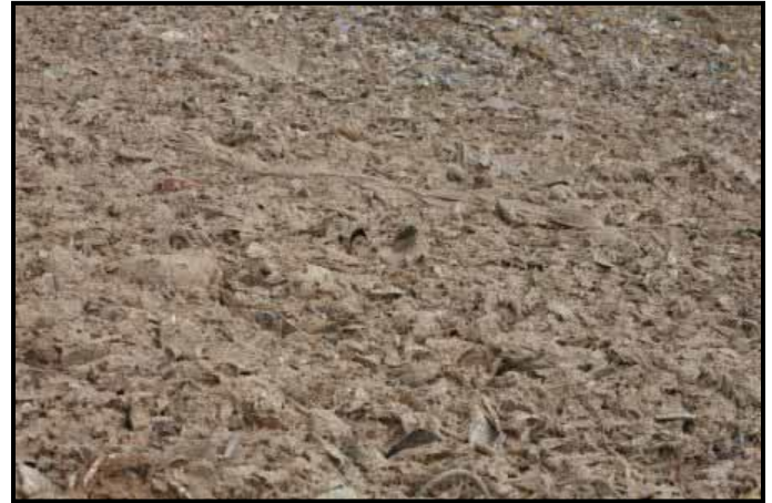
Example of proper application of Topcoat
