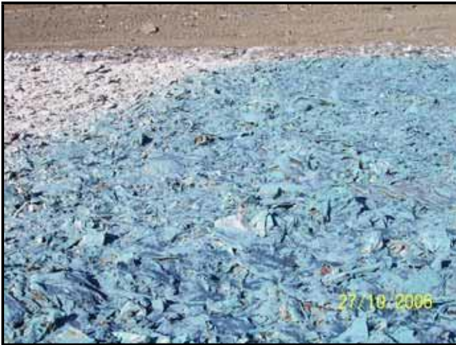
Example of proper application of ConCover
