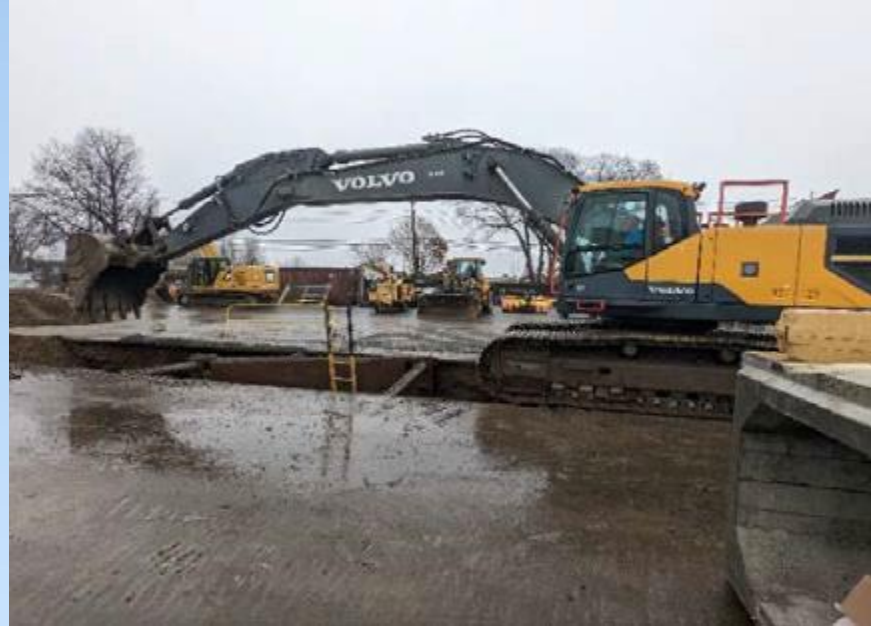
Backfilling trench after installing box culvert at DPW
