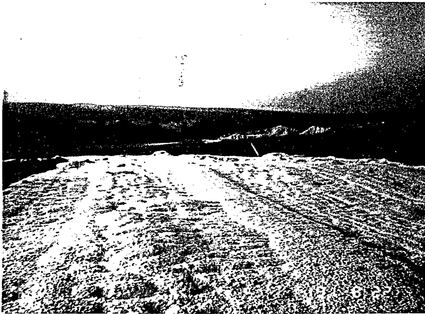
Figures. RUSMAR® foam immediately after application of a 6-in. (15-cm) thick layer.
