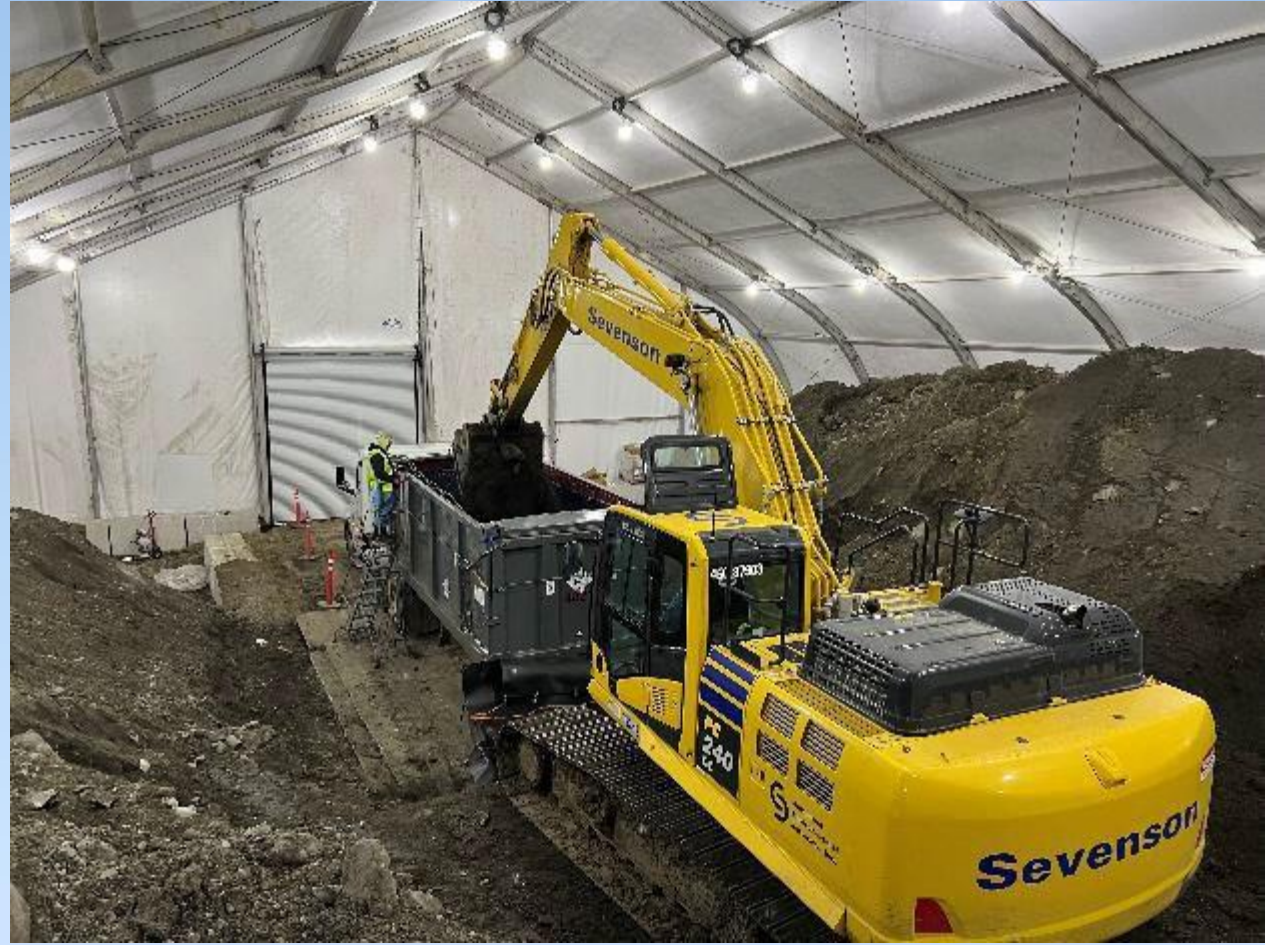
Loading PHC Material for Off-Site Disposal
