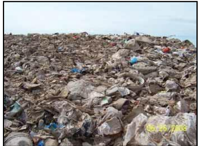
Example of inadequate application of cover material
