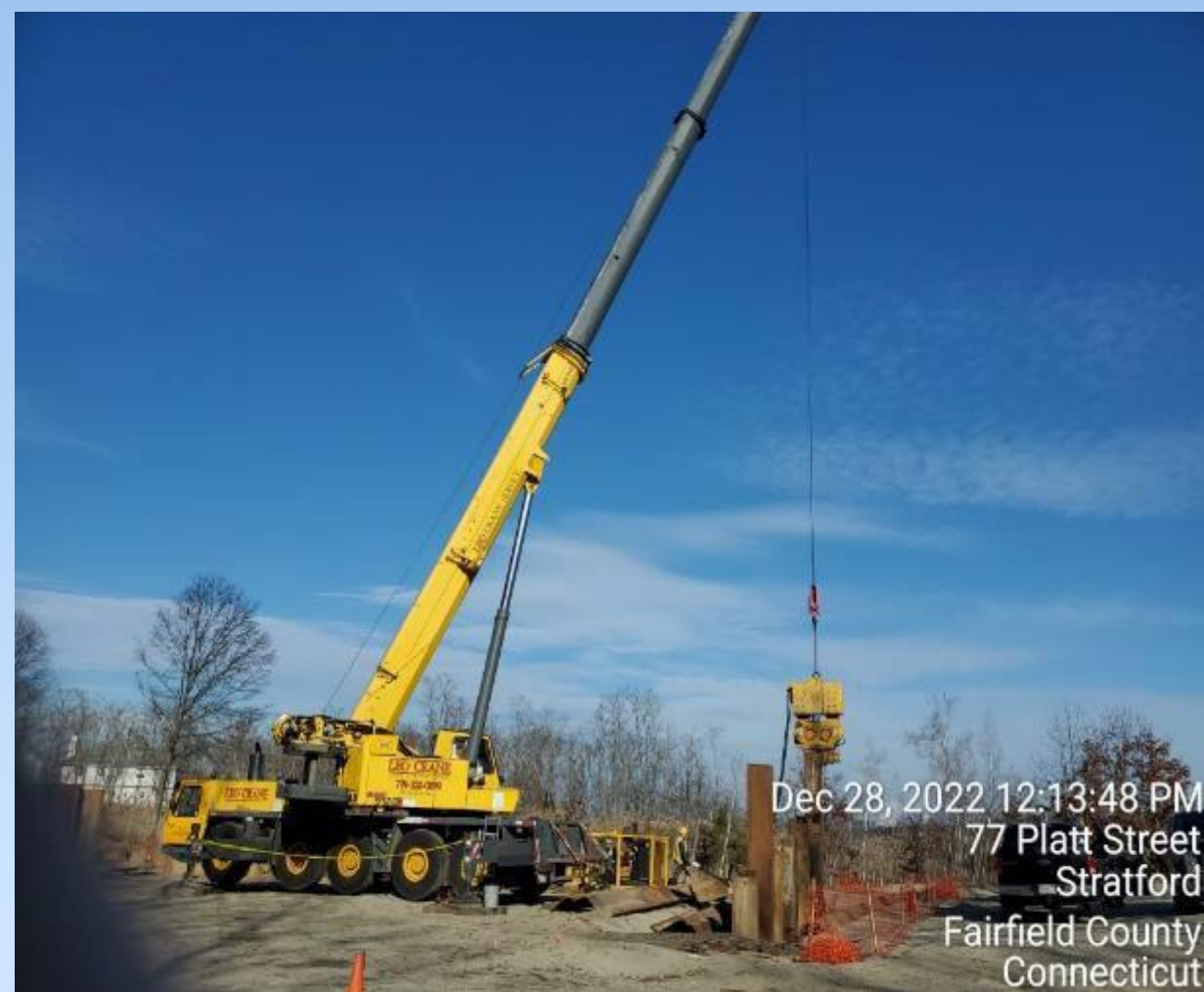
Sheet pile installation
