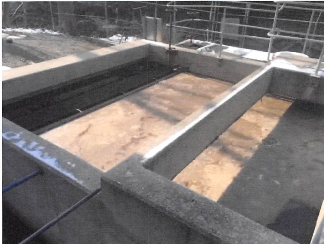
1/31/18 – Clarifier with broken flights
