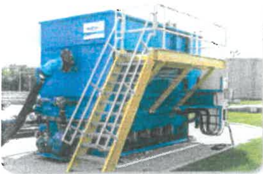
An AquaPrime™ system operating at a municipality for primary treatment.
