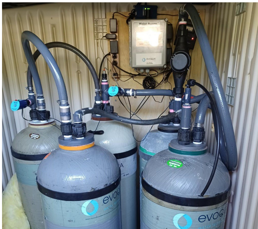
Figure 1. DI Water System
