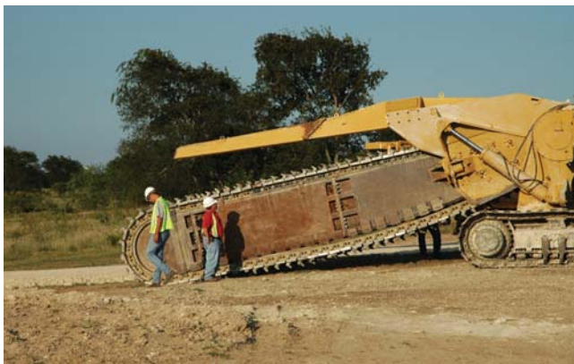
Trenching Machine Used in Biowall Construction
