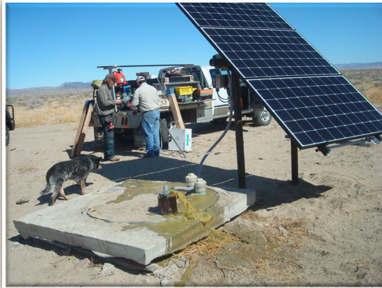
Solar Power for Well Pump
