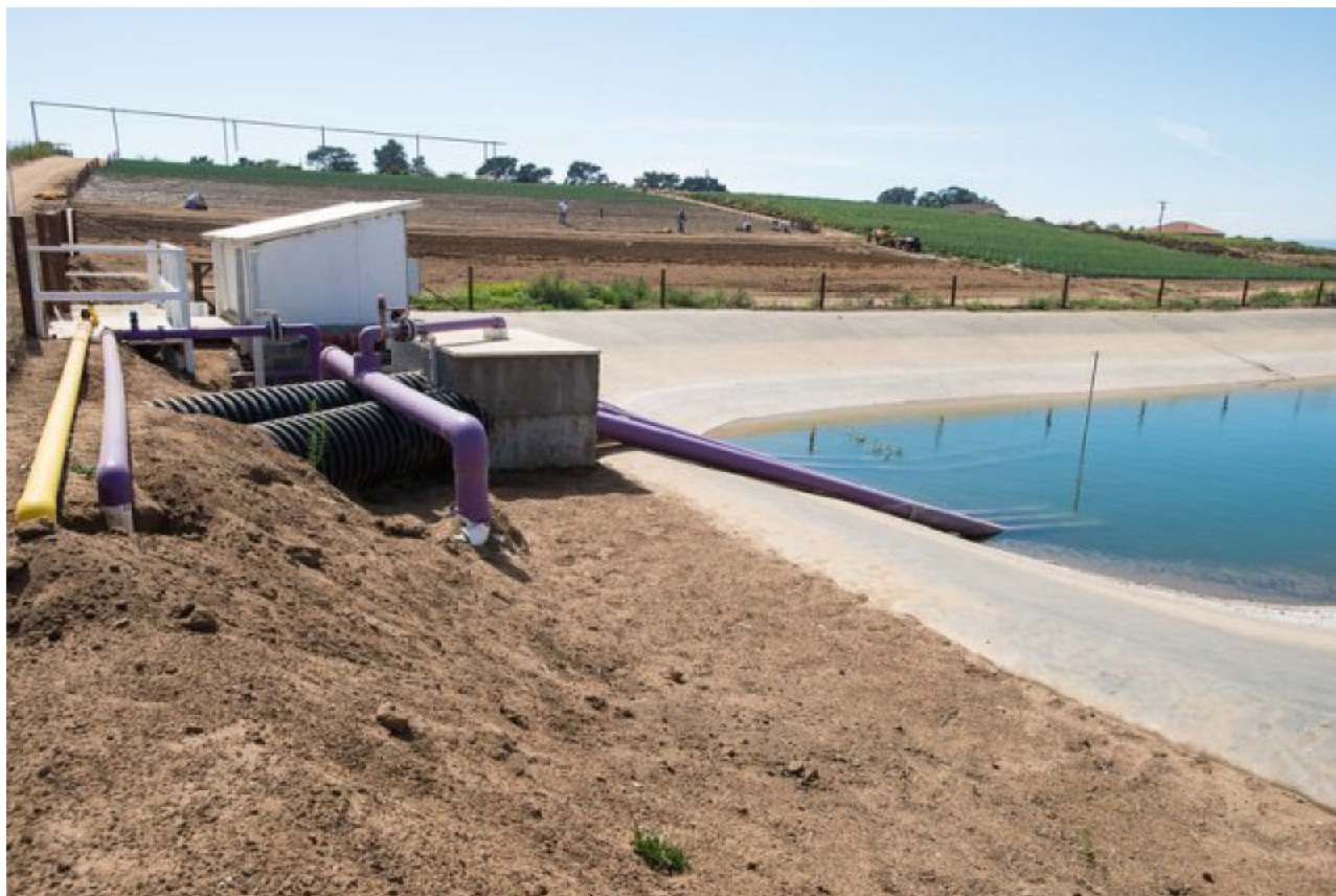
Figure 31. An irrigation tailwater return system in California collects rainwater and treated reclaimed water in a plastic-lined pond, then pumps water to be used for irrigation of fields and greenhouse crops. Photo by U.S. Department of Agriculture.
