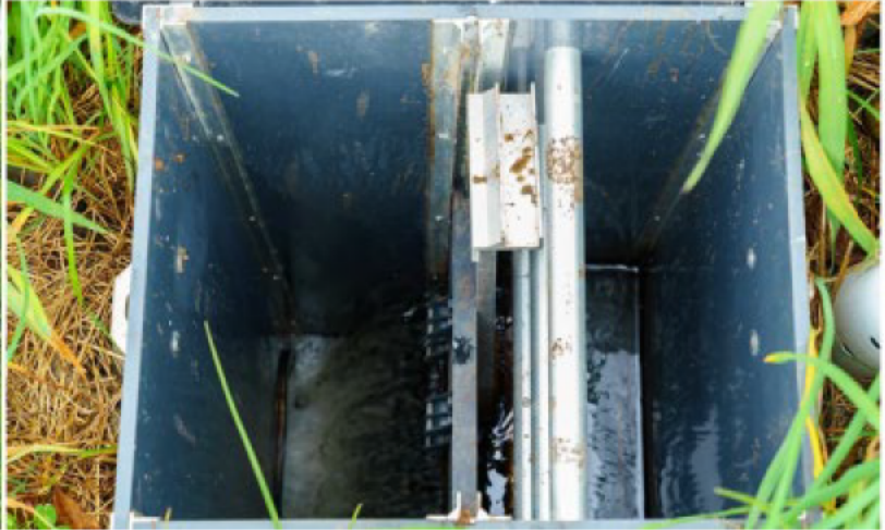
Figure 33. Moving boards inside a water control structure in a wetland in Indiana allow for control of the water level and reduce flooding. Photos by U.S. Department of Agriculture.
