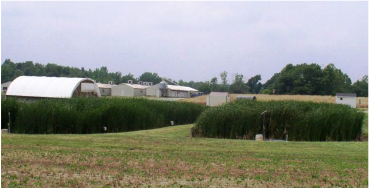
Figure 28. Constructed wetlands on a farm collect runoff from fields. Photo by U.S. Department of Agriculture.
