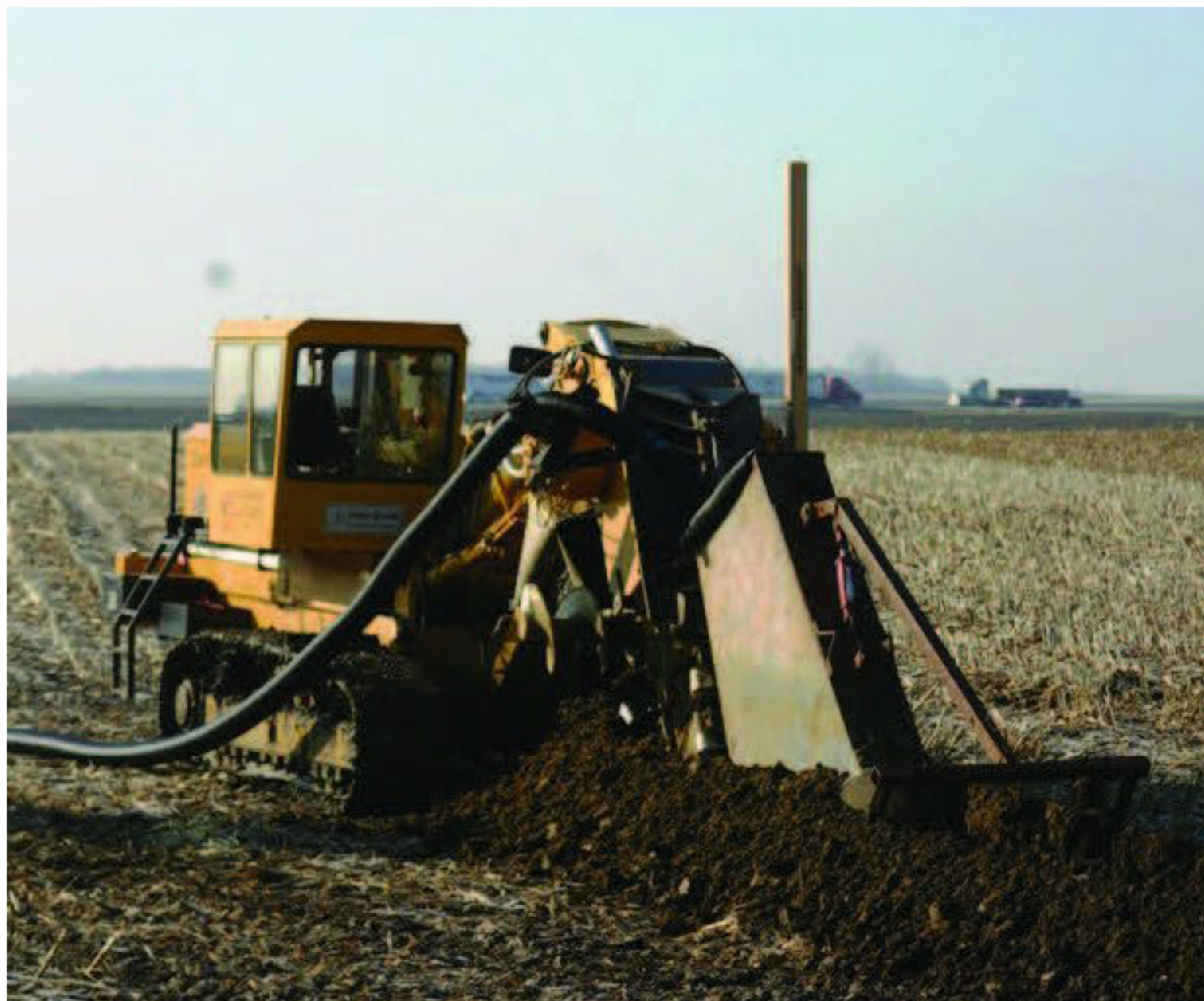
Figure 36. Installation of a subsurface drain. Plastic pipes laid underneath the field carry excess water off the field, either to a controlled or non-controlled water outlet. Photo by U.S. Department of Agriculture.
