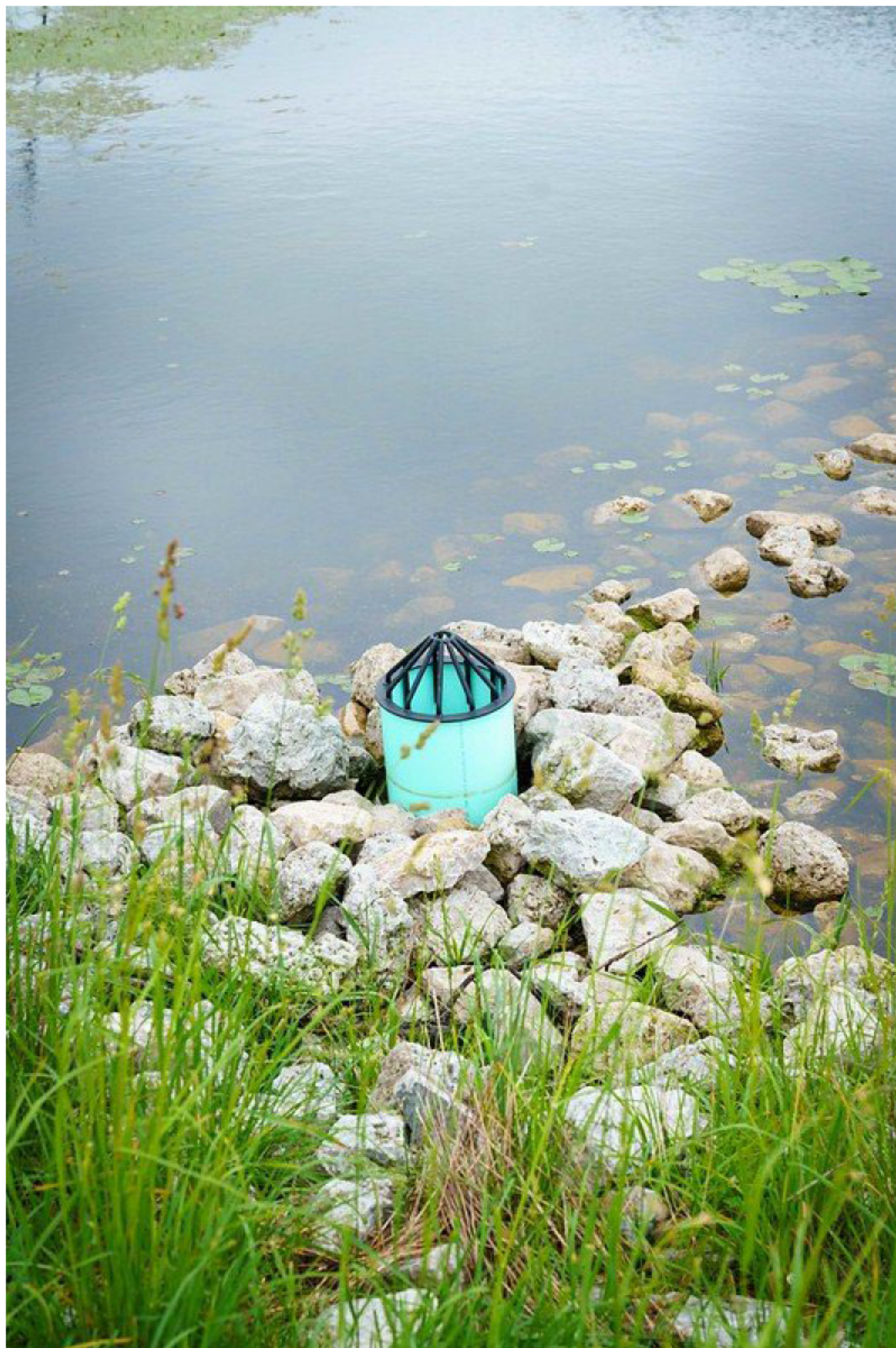
Figure 35. A water control structure in a pond controls water levels by draining excess water. Photo by U.S. Department of Agriculture.
