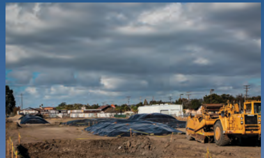
Contaminated soil is removed at the 4.5-acre site that is now the Rumrill Sports Complex.
