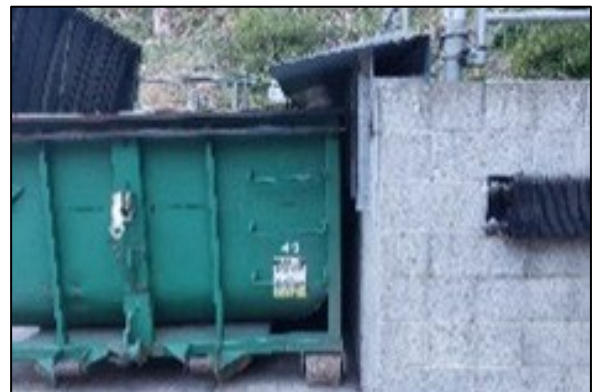
Flaps prevent things falling into the space between container and wall.
