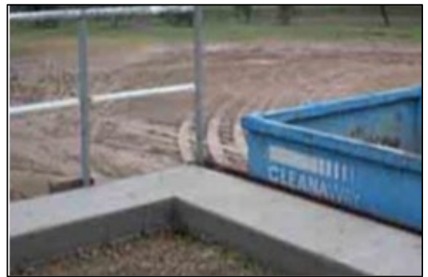
Box placement above the surface reduces the risk of falling.
