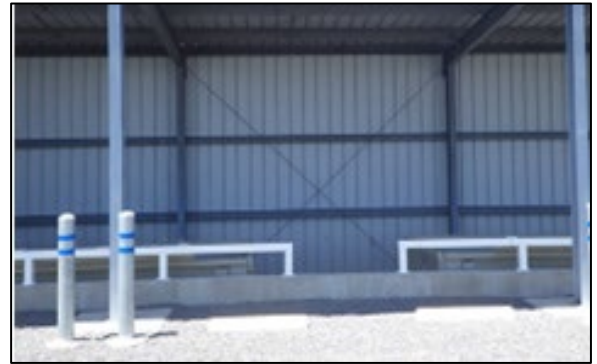
Safety barriers can deter an accidental fall to the lower grade.
