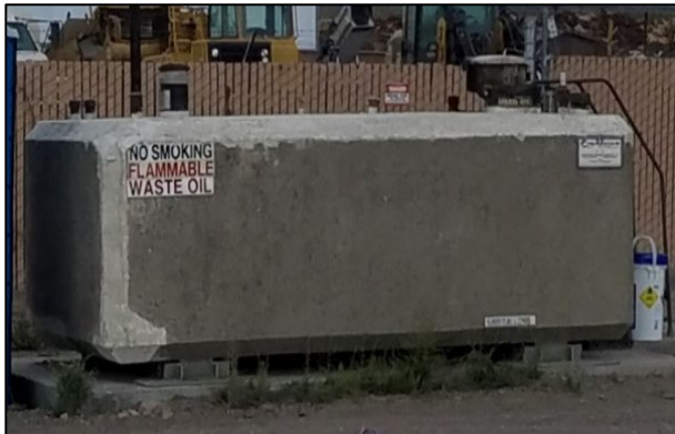
Aboveground tanks for used oil collection.
