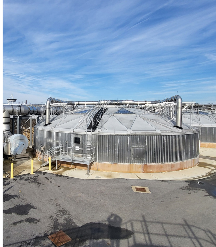
Newly constructed gravity thickeners at the Blue Plains water treatment plant
