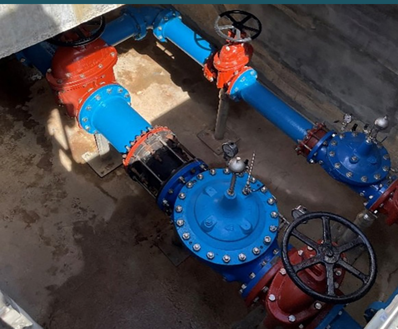
One of the nine newly installed PRV's
