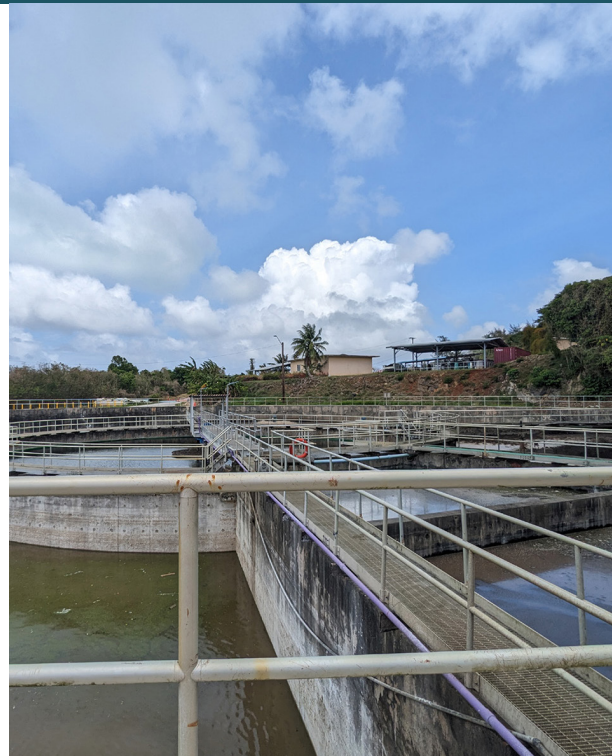
The newly-installed clarifier at the CUC Wastewater Treatment Plant
