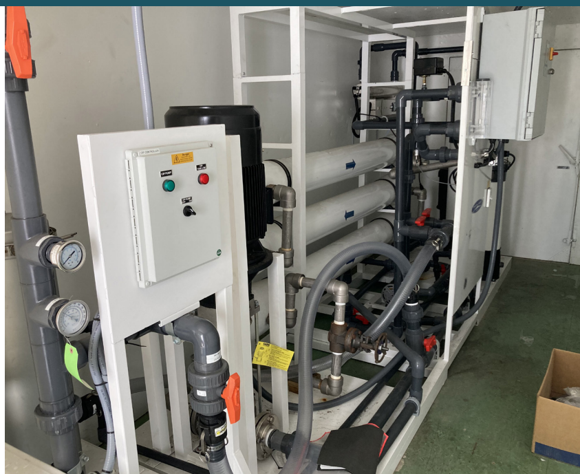
The newly installed reverse osmosis drinking water plant at Coakley Bay Condominium
