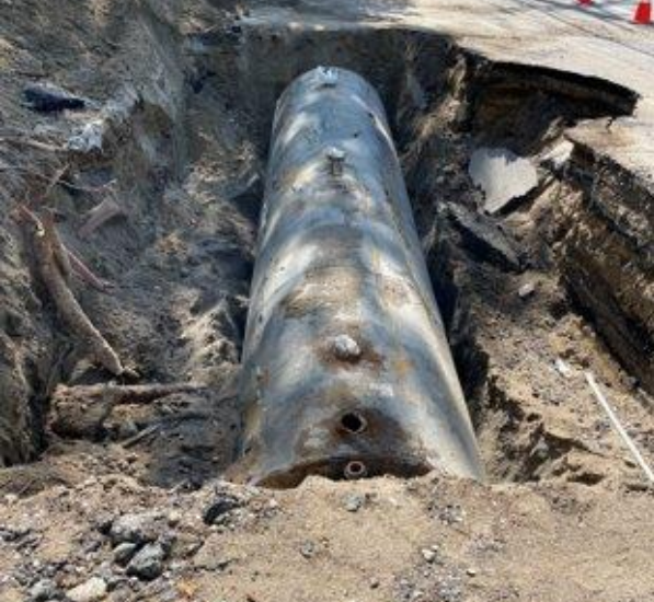
One 4,000-gallon gasoline tank removed from the site in May 2023.
