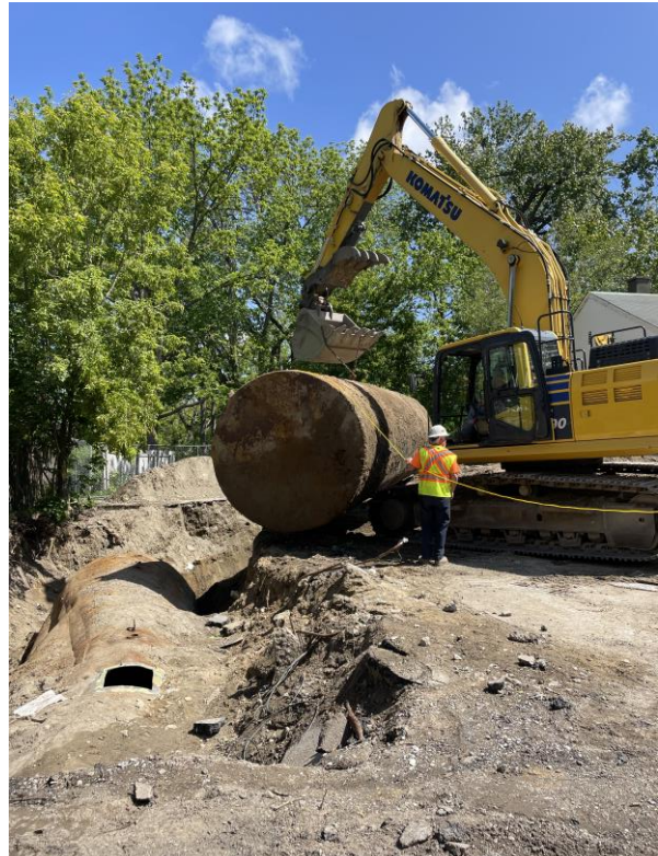
Two 10,000-gallon gasoline tanks being removed from the site in May 2023.
