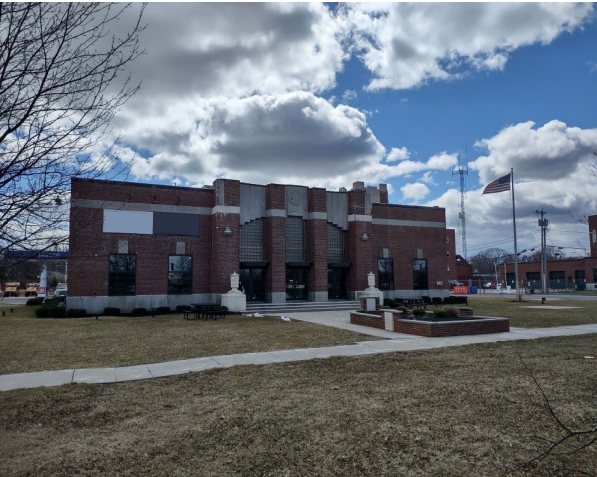
View of redeveloped Maine National Guard Armory. (Photo credit: City of South Portland)
