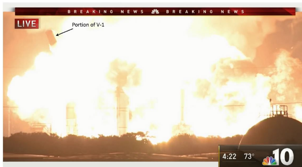
Figure 18: Video still of one of the 2019 Philadelphia refinery explosions, showing a 19-ton projectile (labeled “Portion of V-1”) that flew more than 2,000 feet 191
