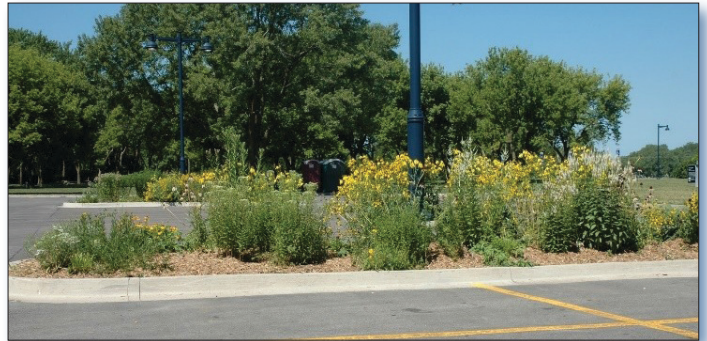
Bioretention cells installed in parking lot to treat runoff.
