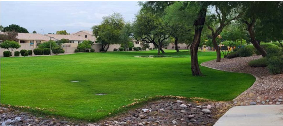
Retention/Detention basin with drywells used as a flood control strategy to capture and direct stormwater for recharge in Chandler, AZ. Photo taken by Tianfang Xu
