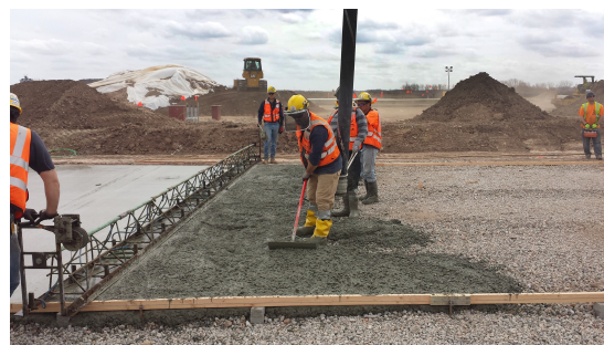
Construction workers lay gravel over cement soil cap in Woodbridge, NJ.
