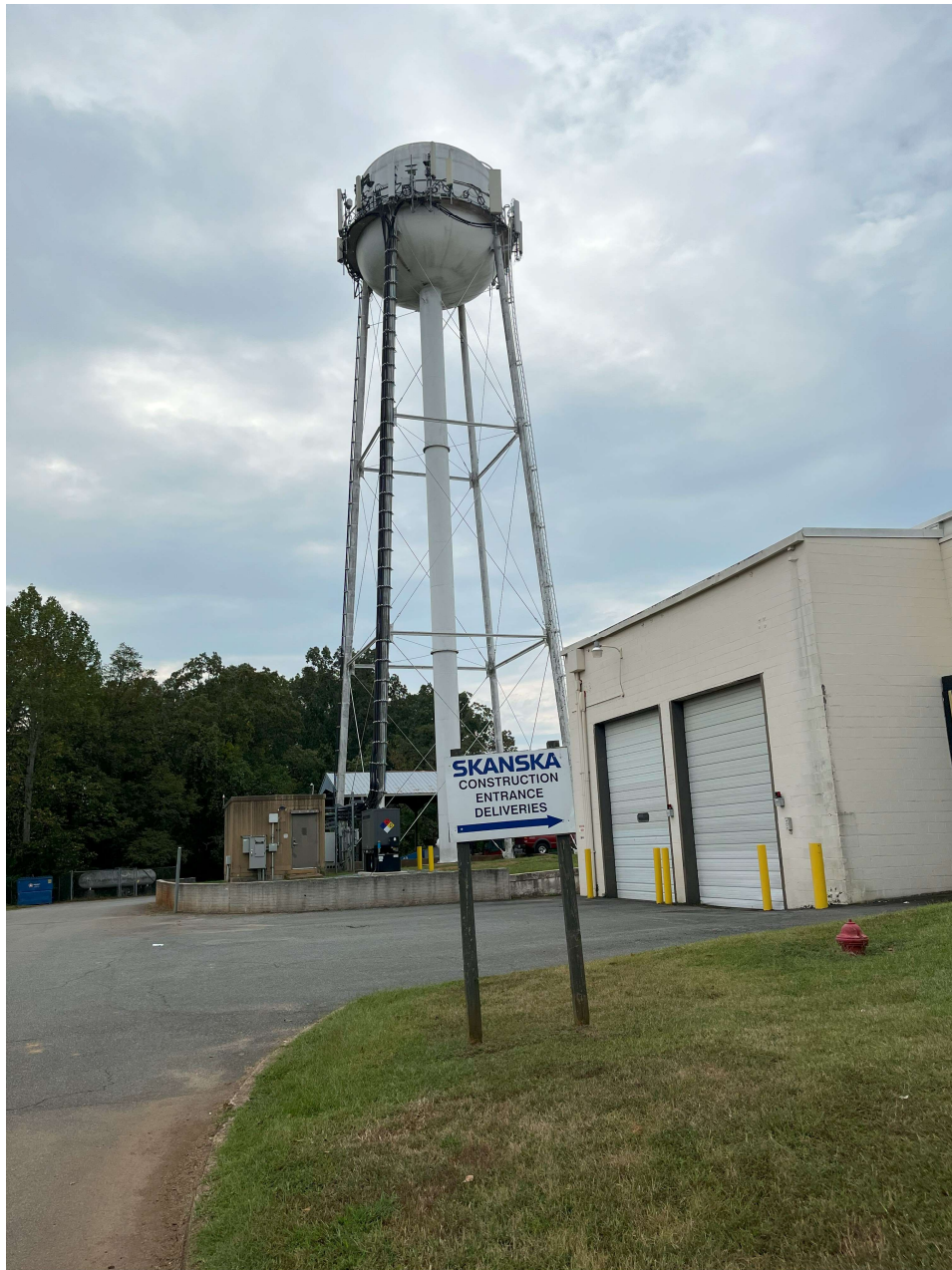
Southeast corner of facility including water tower – looking south
