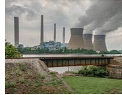
New Power Plant
