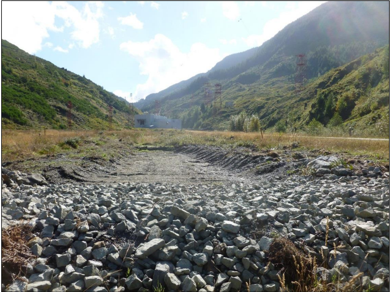
Figure 3. Southeasterly view of the new infiltration pond installed upstream of Outfall 067.
