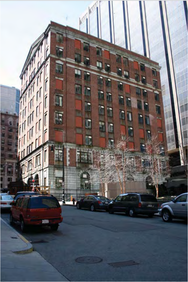
Somerset Street (east) and north facades
