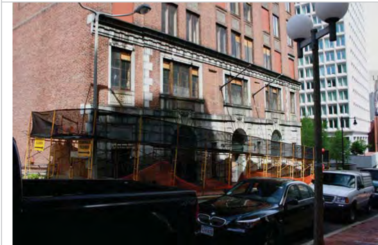
Ground floor detail – Somerset Street
