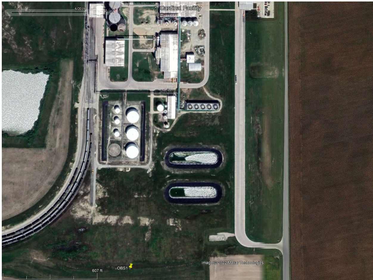
Figure 4. Ethanol facility and OBS1 location
