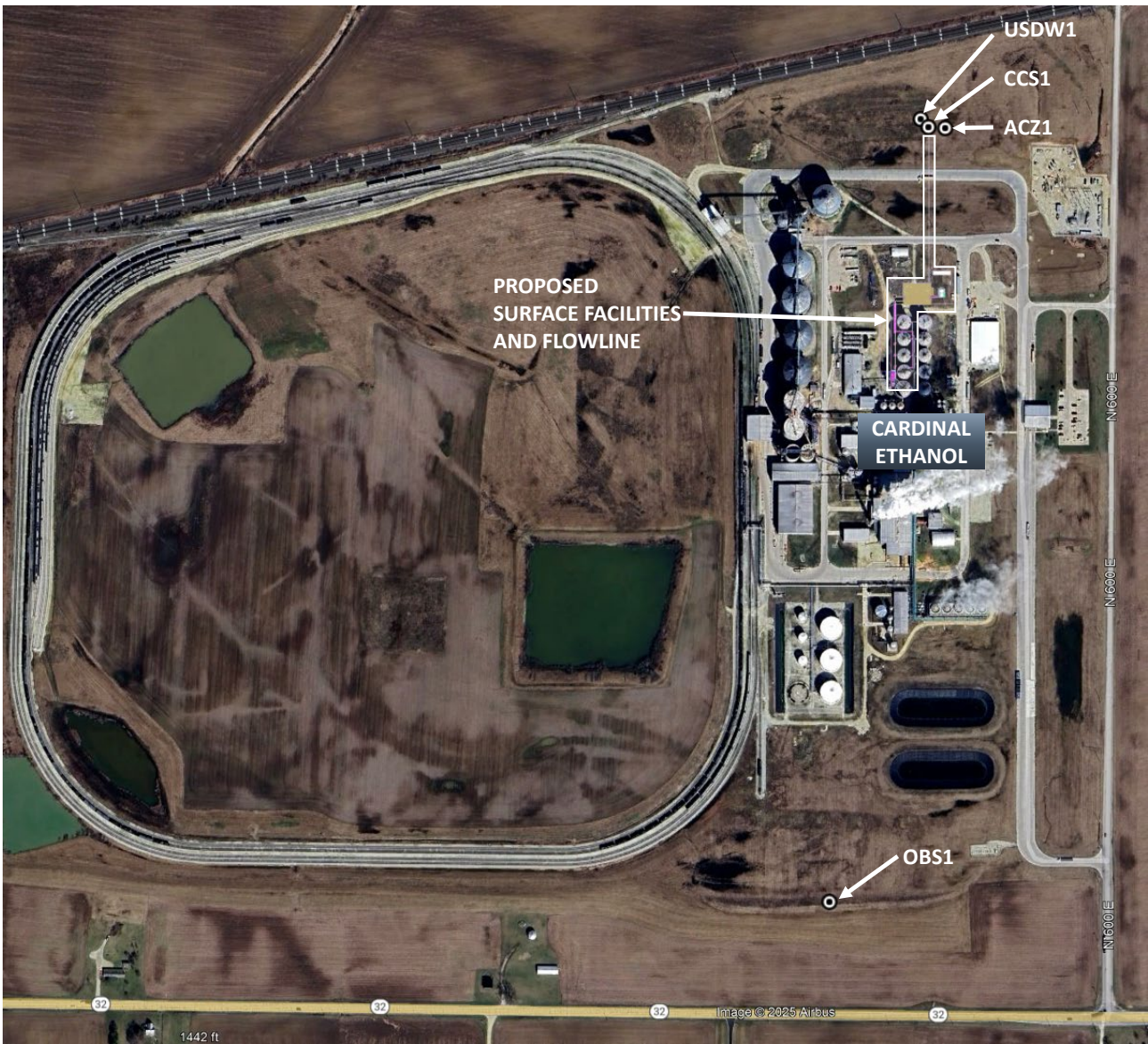
Figure 2. Cardinal Ethanol facility and associated CCS related equipment.
