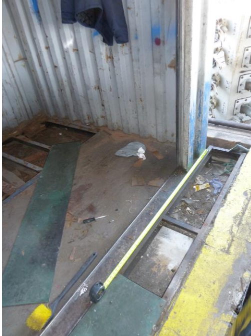
Figure #7 Concrete Sample Location – East Containment Area (North Side)
