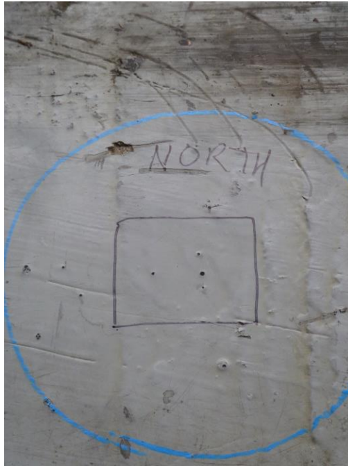
Figure #15 Wipe Sample Location – Non-PCB Containment Area Floor – North
