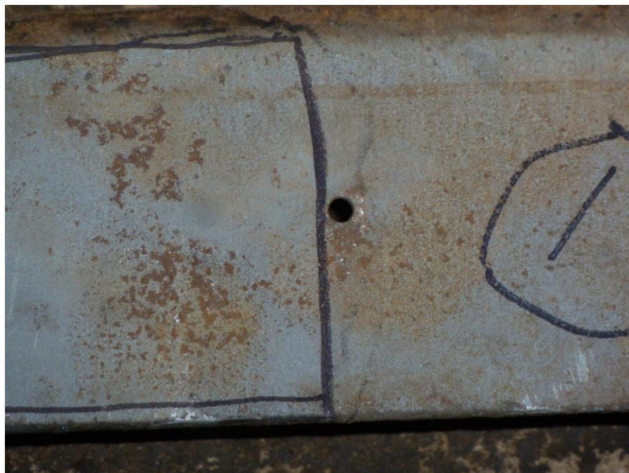
Figure #11 Wipe Sample Location – Containment Floor Sample #1
