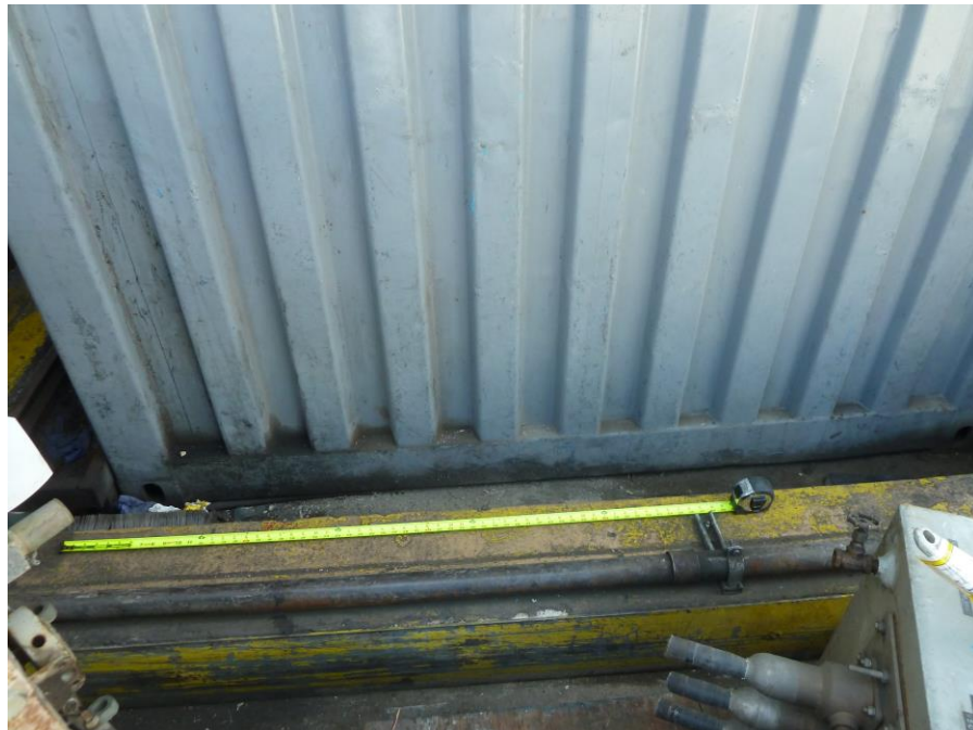
Figure #10 Concrete Sample Location – West Containment Area
