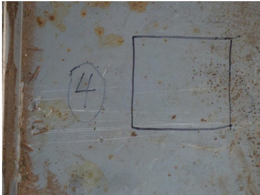
Figure #14 Wipe Sample Location – Containment Floor Sample #4
