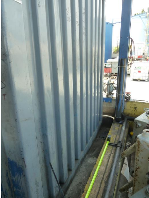
Figure #9 Concrete Sample Location – North Containment Area
