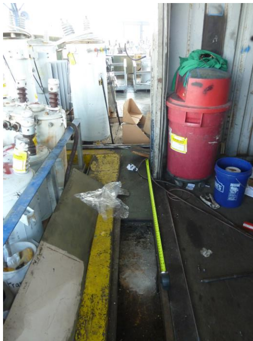
Figure #6 Concrete Sample Location – East Containment Area (South Side)
