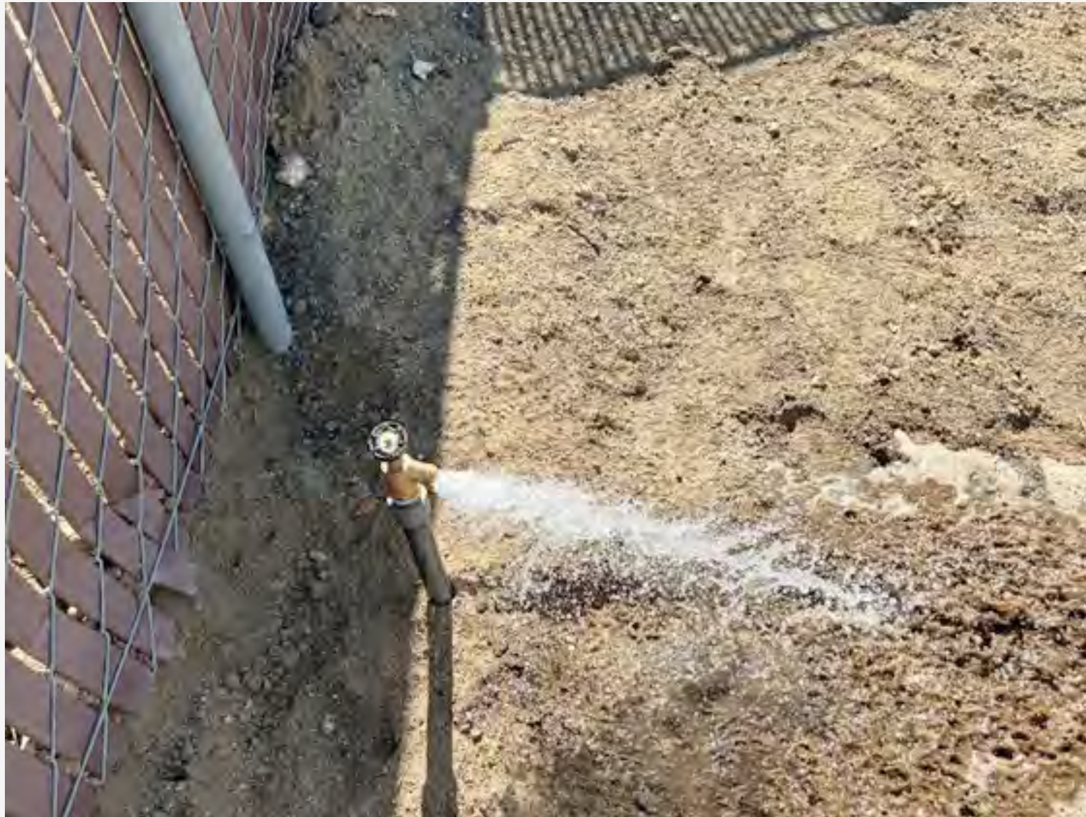
Installed 9 hose bibs, providing adequate water access across the site
