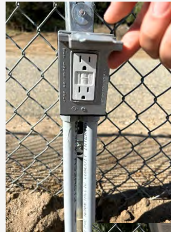
Installed 8 dual port 120 volt outlets around the perimeter.
