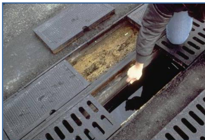
Figure 5. Ensuring the long-term maintenance of sand filters, swales, bioretention facilities, and other BMPs is a critical component of a municipal stormwater management program.
