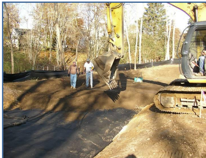
Figure 4. As an example of a priority retrofit taken to final design and construction, this shows the installation of a bioretention facility at a nature center in Massachusetts.
