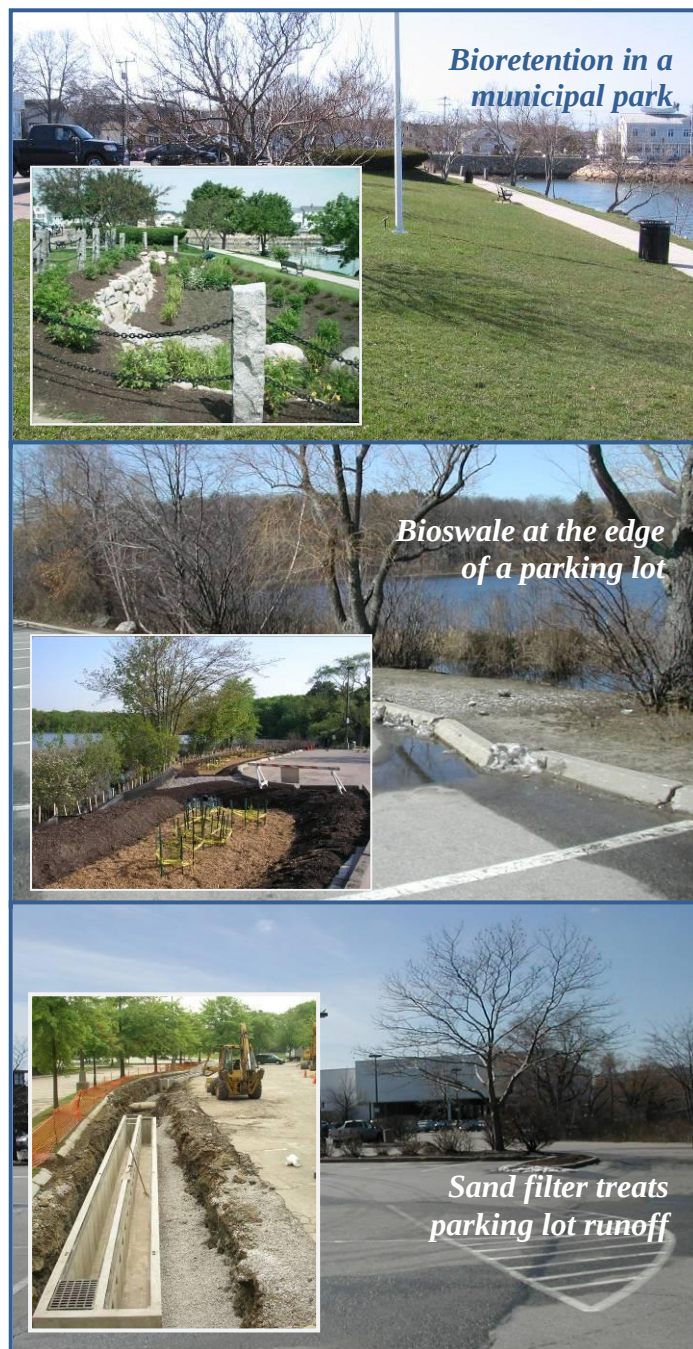
Figure 1. Structural retrofits such as the bioretention, bioswale, and sand filter shown here can be used to capture, treat, and/or infiltrate unmanaged runoff. Public open space and large parking lots are common retrofit locations.
