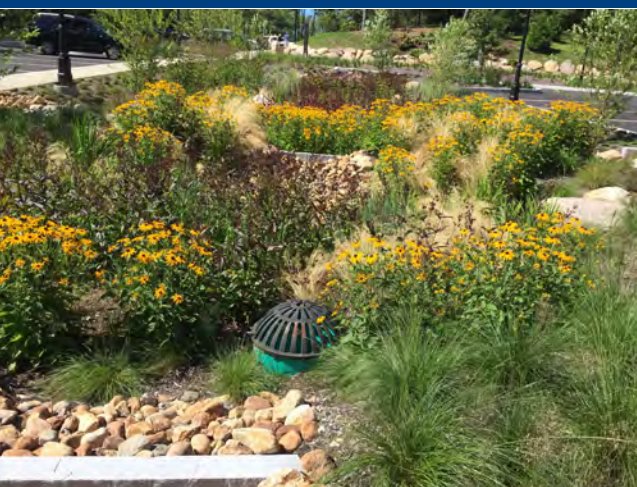
Bioretention Basin (Credit: HW)
