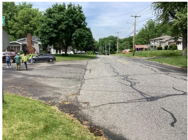
Grandview Street at Hillside Avenue
