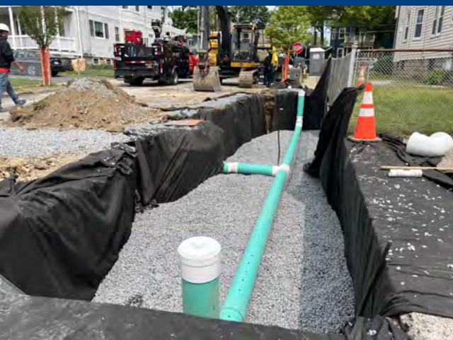
Gravel Reservoir/Underdrain of Tree Trench
