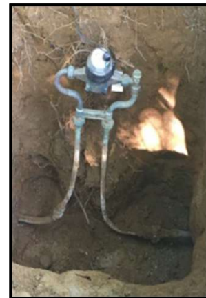
Example of Meter Pit and Service Lines Source LSLR Collaborative 2018
