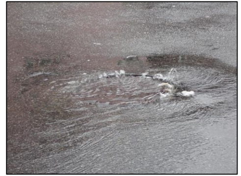
An SSO flows on to a city street.
