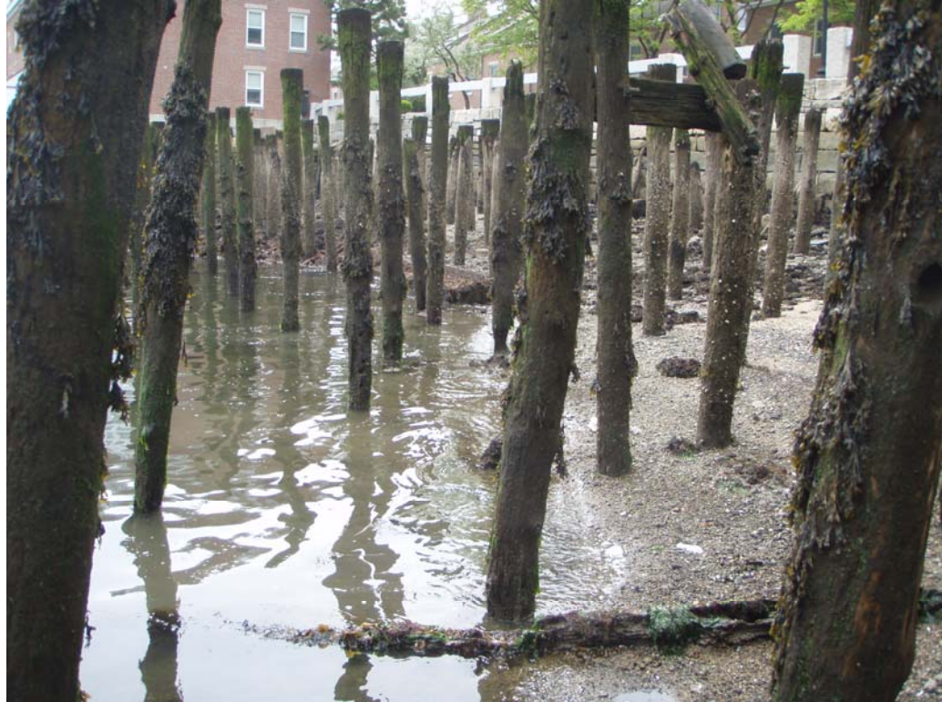
Figure 5 – Beach Area and Pile Field
